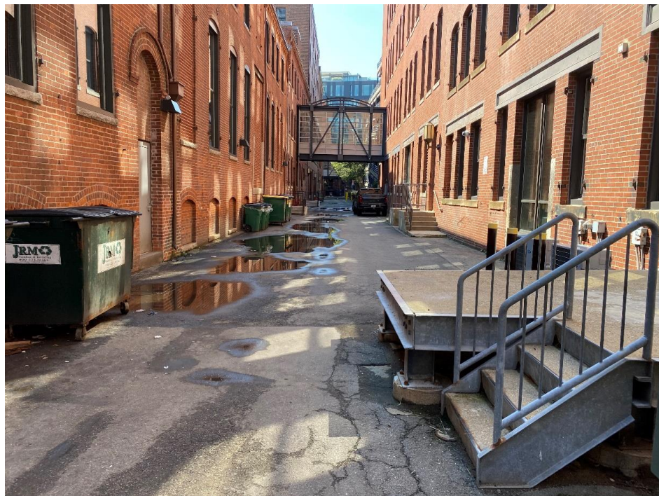
Picture 4: Loading dock in private alley way behind building.
