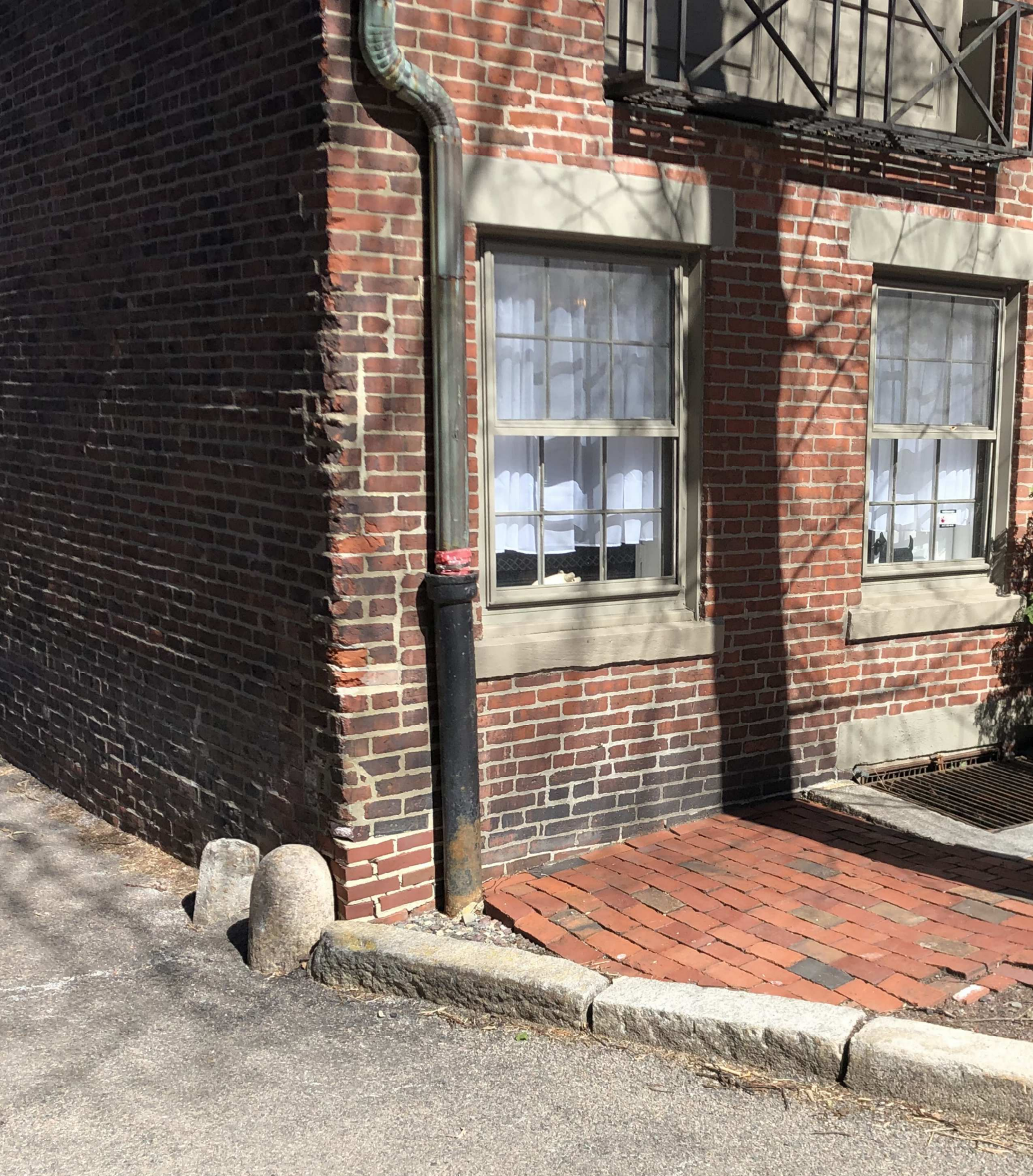
1 River Street Place View of Corner
