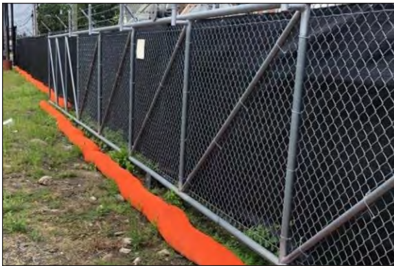
Filtrexx SiltSoxx EXTREME used in rugged conditions.
