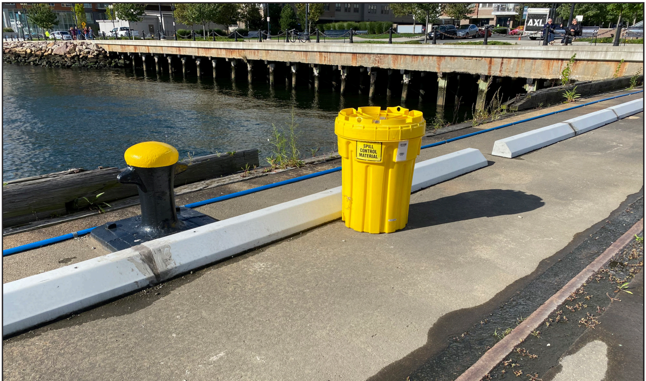
Photograph 4: Curb stop and spill containment.
