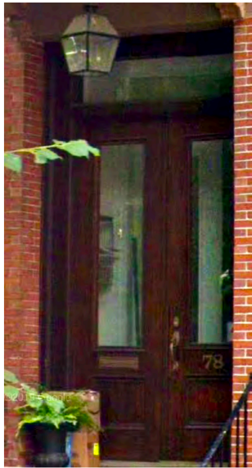
Existing front doors
