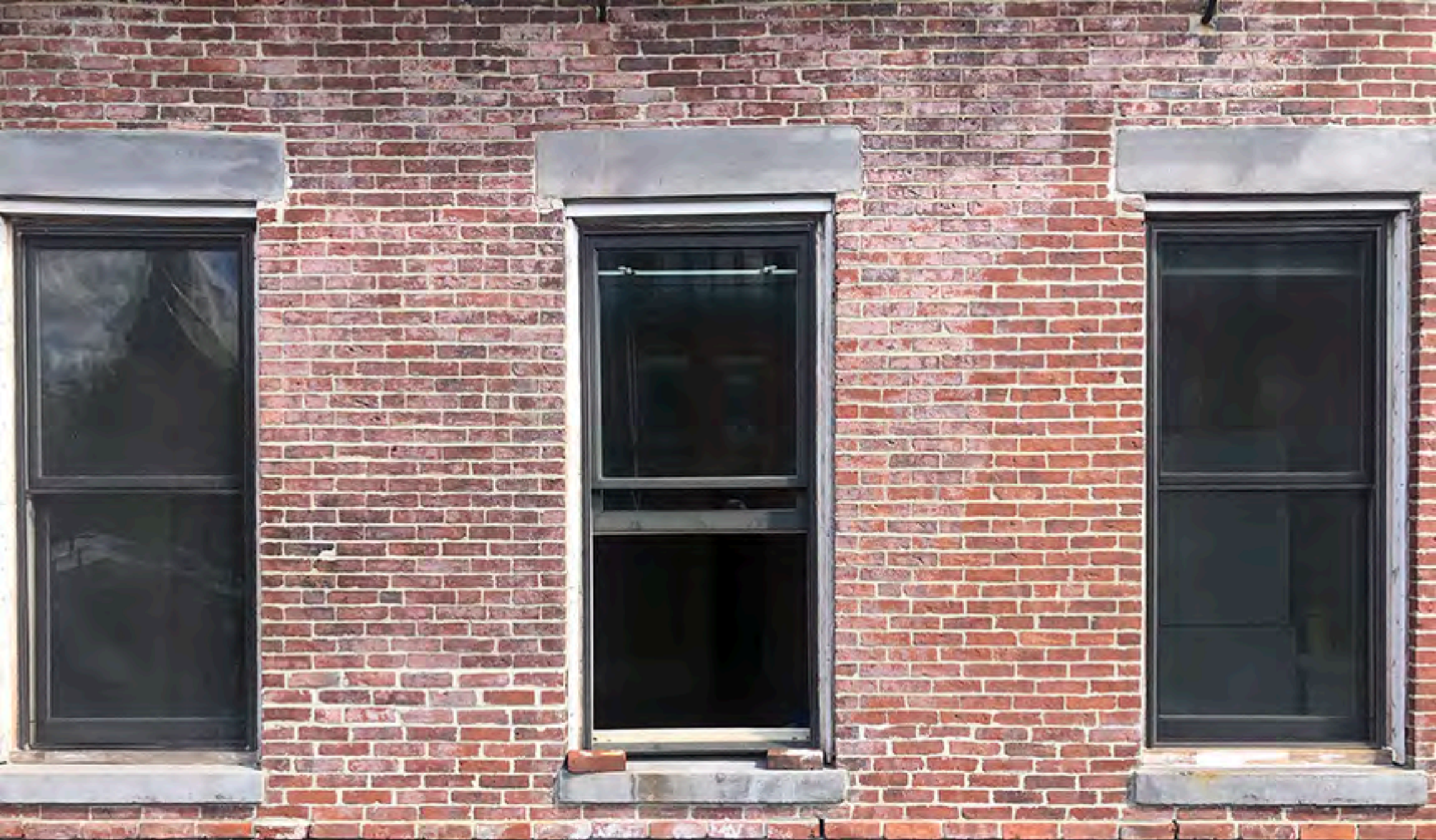
Level 3 rear windows
