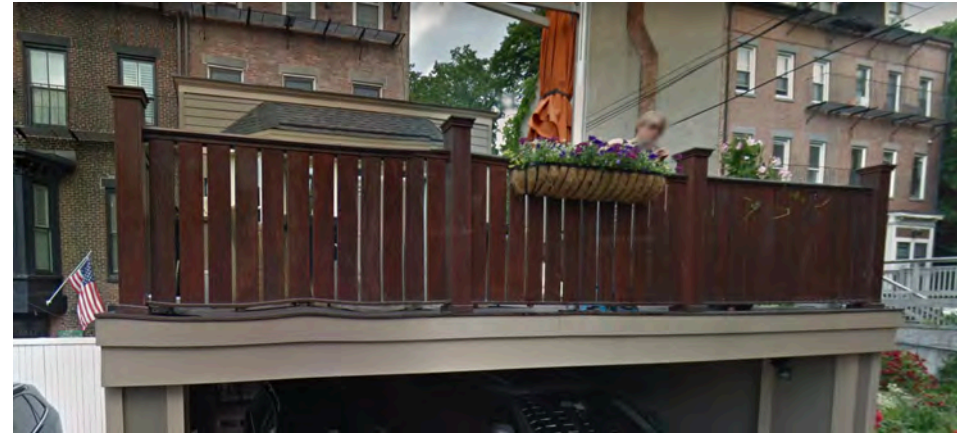
Existing ipe railing on level 2
