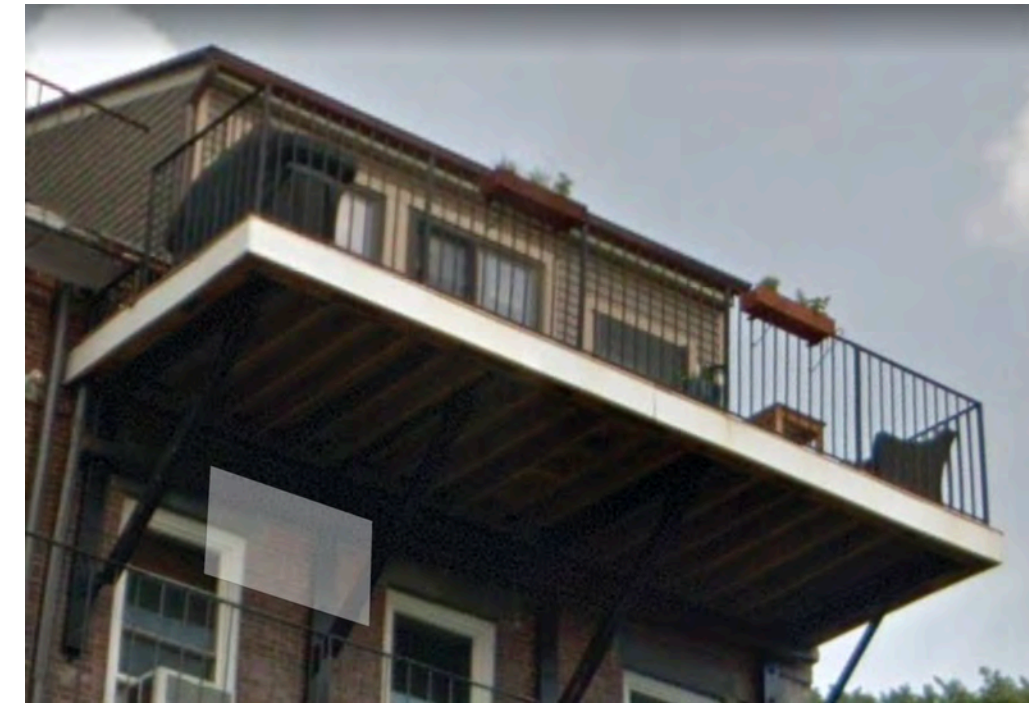
Existing iron railing
