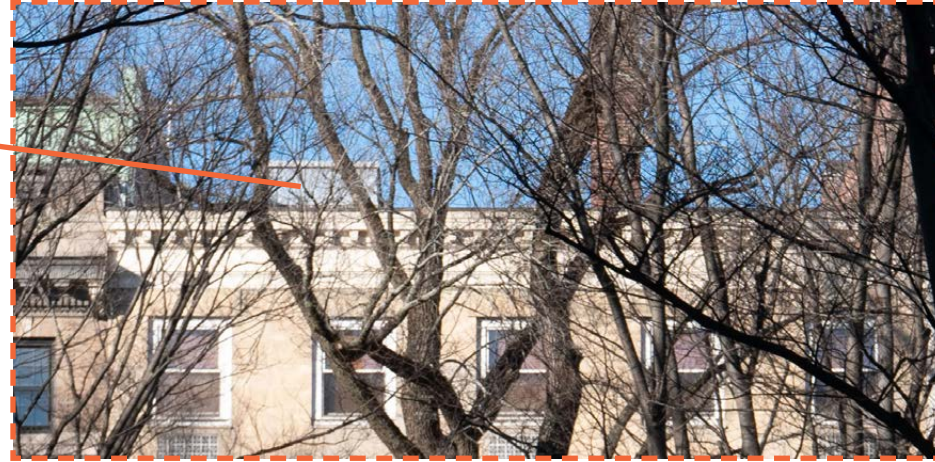
Existing visible elevator head house (to be removed)
