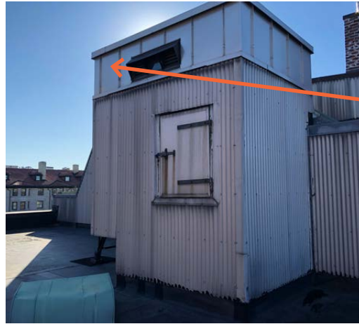
Existing elevator head house, galvanized corrugated and standing seam
