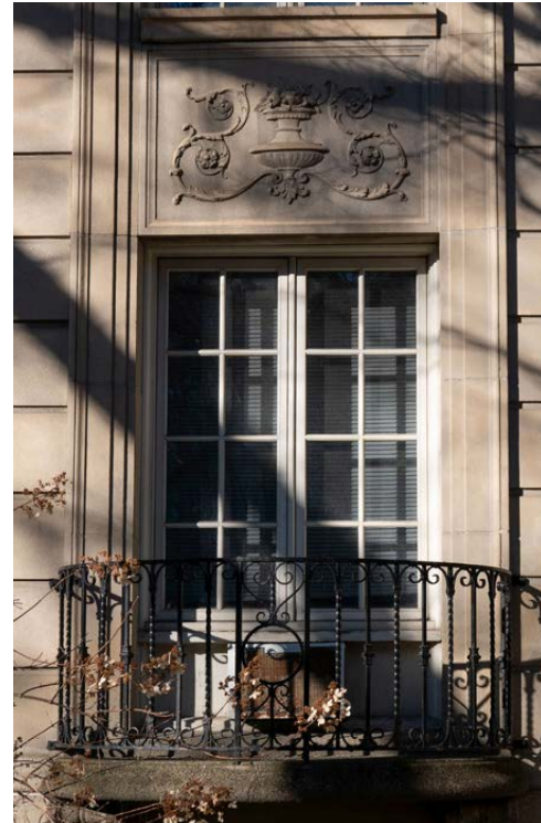
Existing (non-original) casement windows at Level 1
