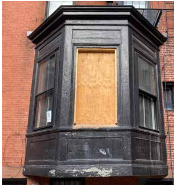
FIRST FLOOR ORIEL WINDOW
