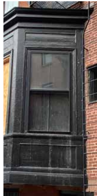
FIRST FLOOR ORIEL WINDOW
