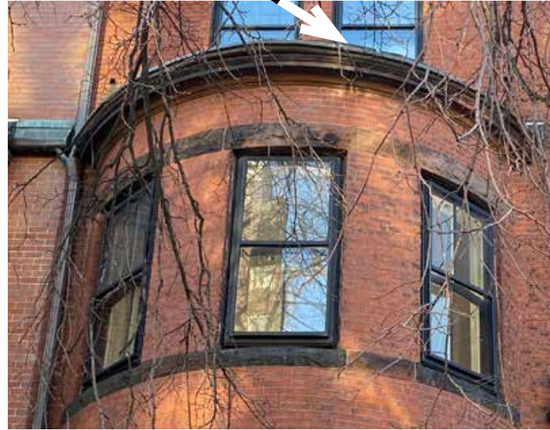
SECOND FLOOR BAY WINDOW
