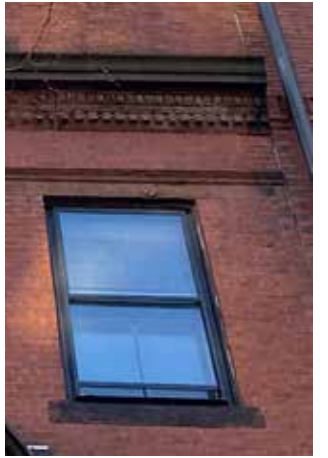
THIRD FLOOR WINDOW
