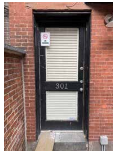
GROUND FLOOR DOOR
