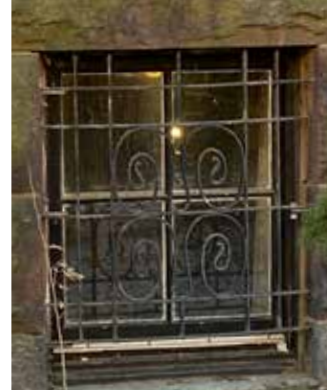
GROUND FLOOR BAY WINDOW
