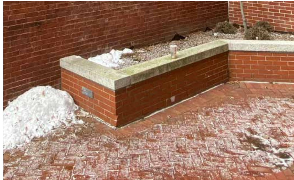
PLANTER AT SIDE (NORTHEAST) FACADE AND NEIGHBOR'S DRIVEWAY
