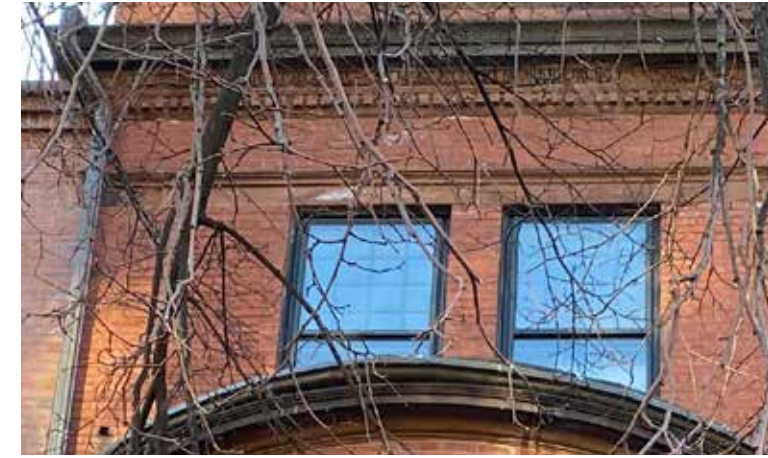
THIRD FLOOR WINDOW
