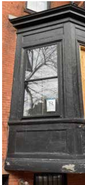
FIRST FLOOR ORIEL WINDOW
