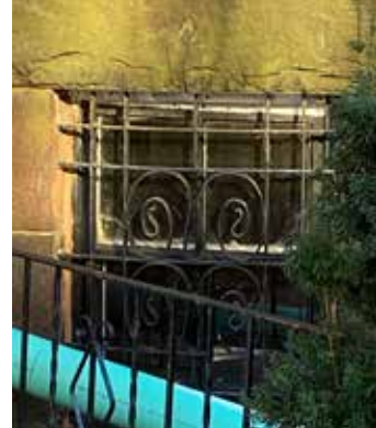
GROUND FLOOR BAY WINDOW
