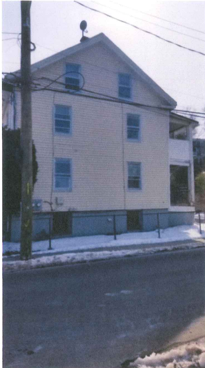
2) Right Side of 104 Jamaica Street
