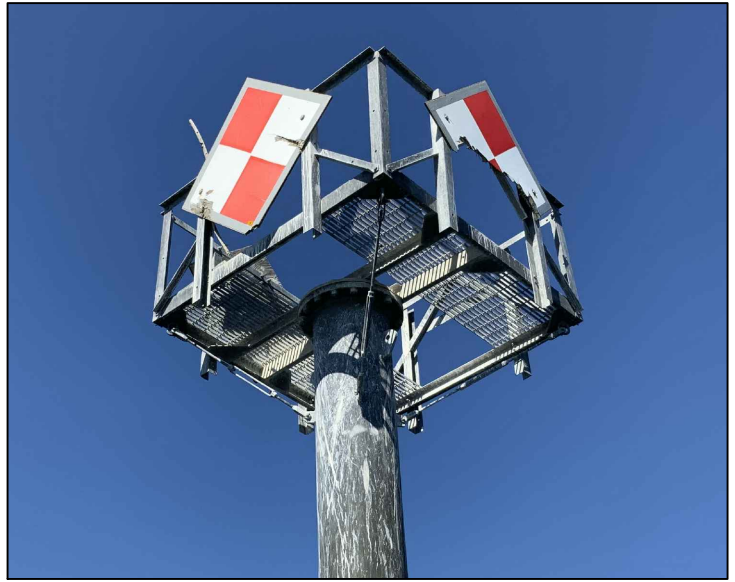
A6 PLATFORM LOOKING NORTHWEST SCALE: NTS
