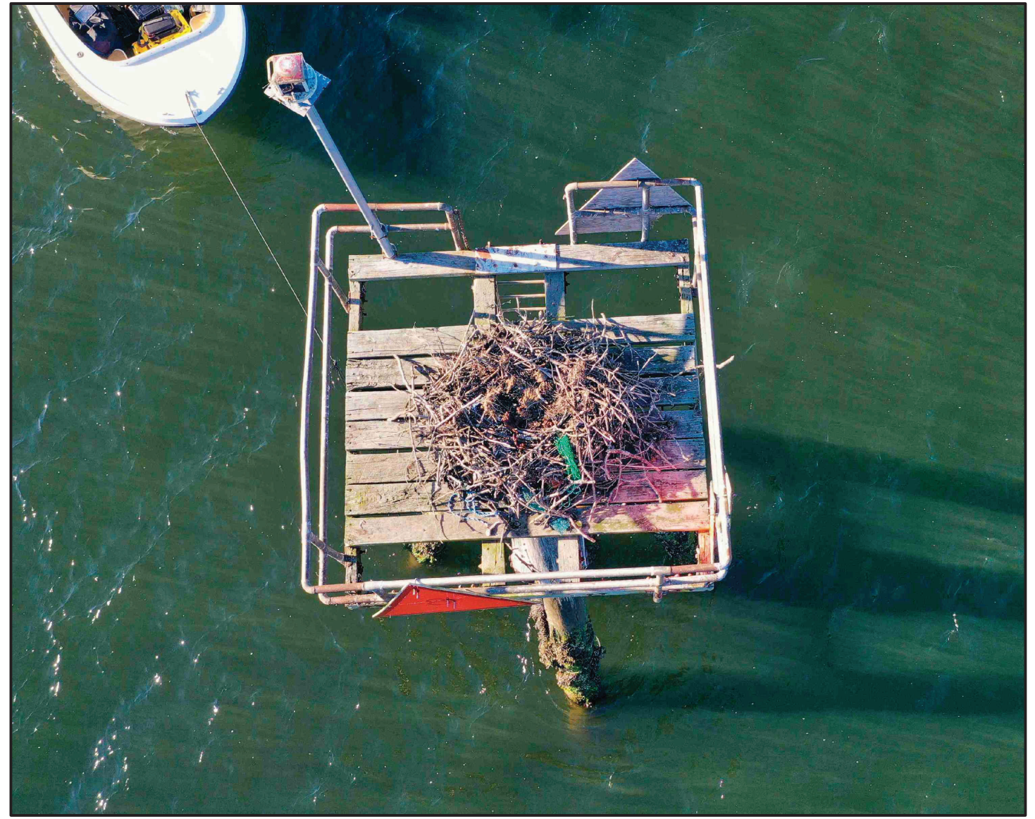
A6 PLATFORM LOOKING NORTH SCALE: NTS
