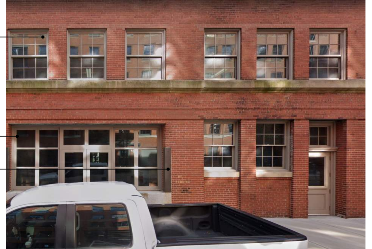
9 CHANNEL CENTER AFTER - RENOVATION (2020 STREET VIEW)
