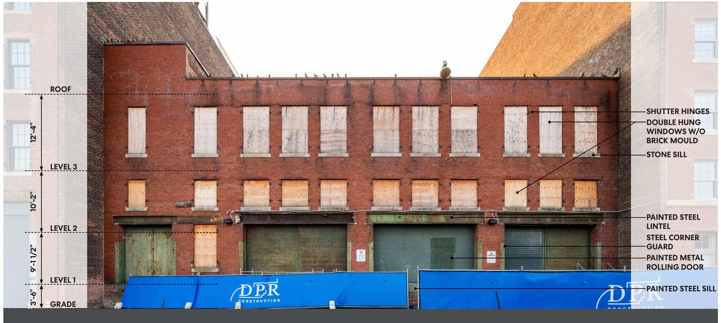
EXISTING FAÇADE - EAST (MEDALLION AVE)
