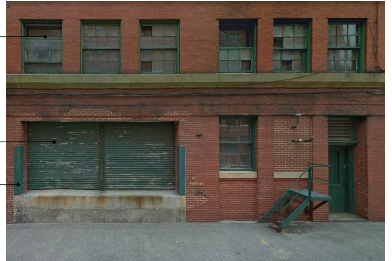
9 CHANNEL CENTER BEFORE RENOVATION (2011 STREET VIEW)
