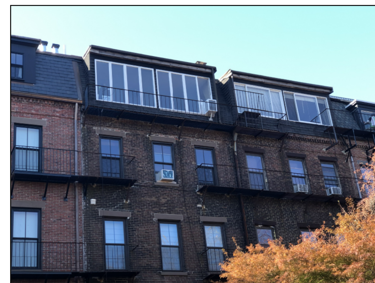
5 VIEW FROM REAR OF BUILDING
