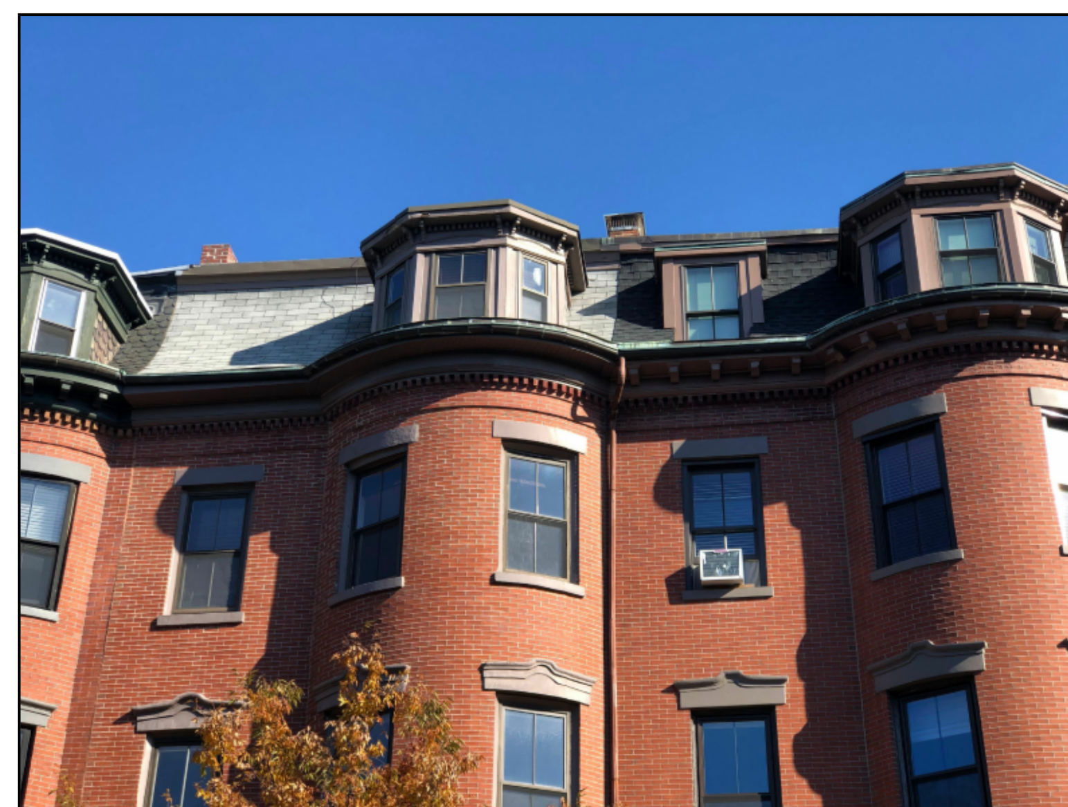
2 VIEW FROM WORCESTER ST.
