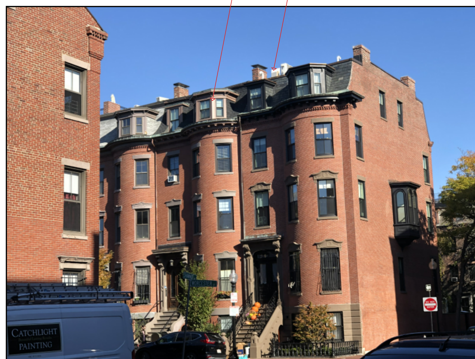
1 VIEW FROM SHAWMUT AVE.
