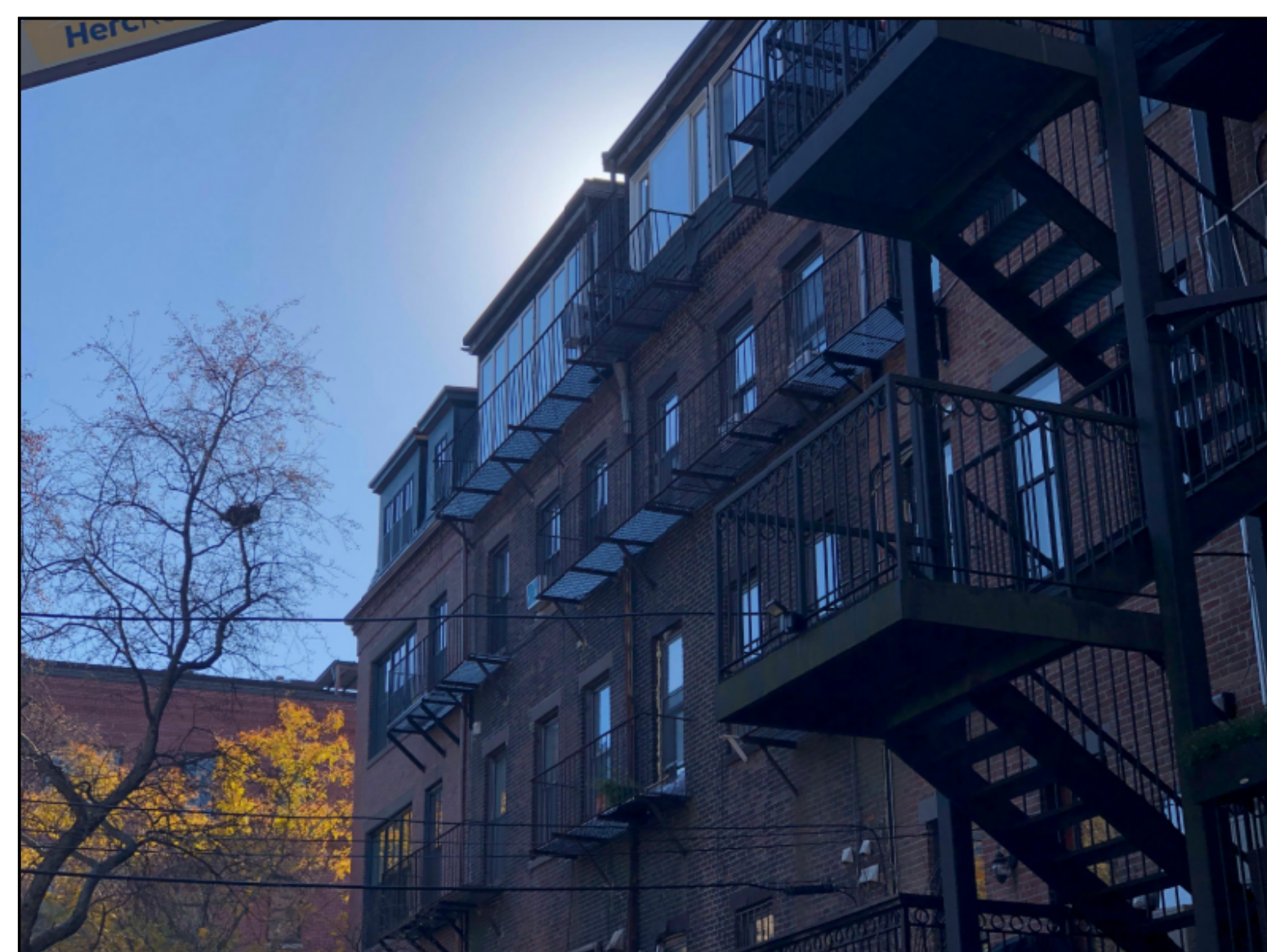
4 VIEW FROM INTERSECTION OF NEWLAND ST. & PUBLIC ALLEY
