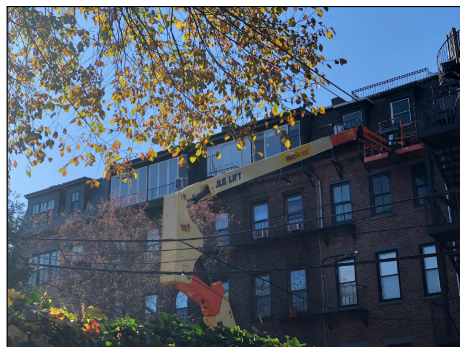
5 VIEW FROM NEWLAND ST.
