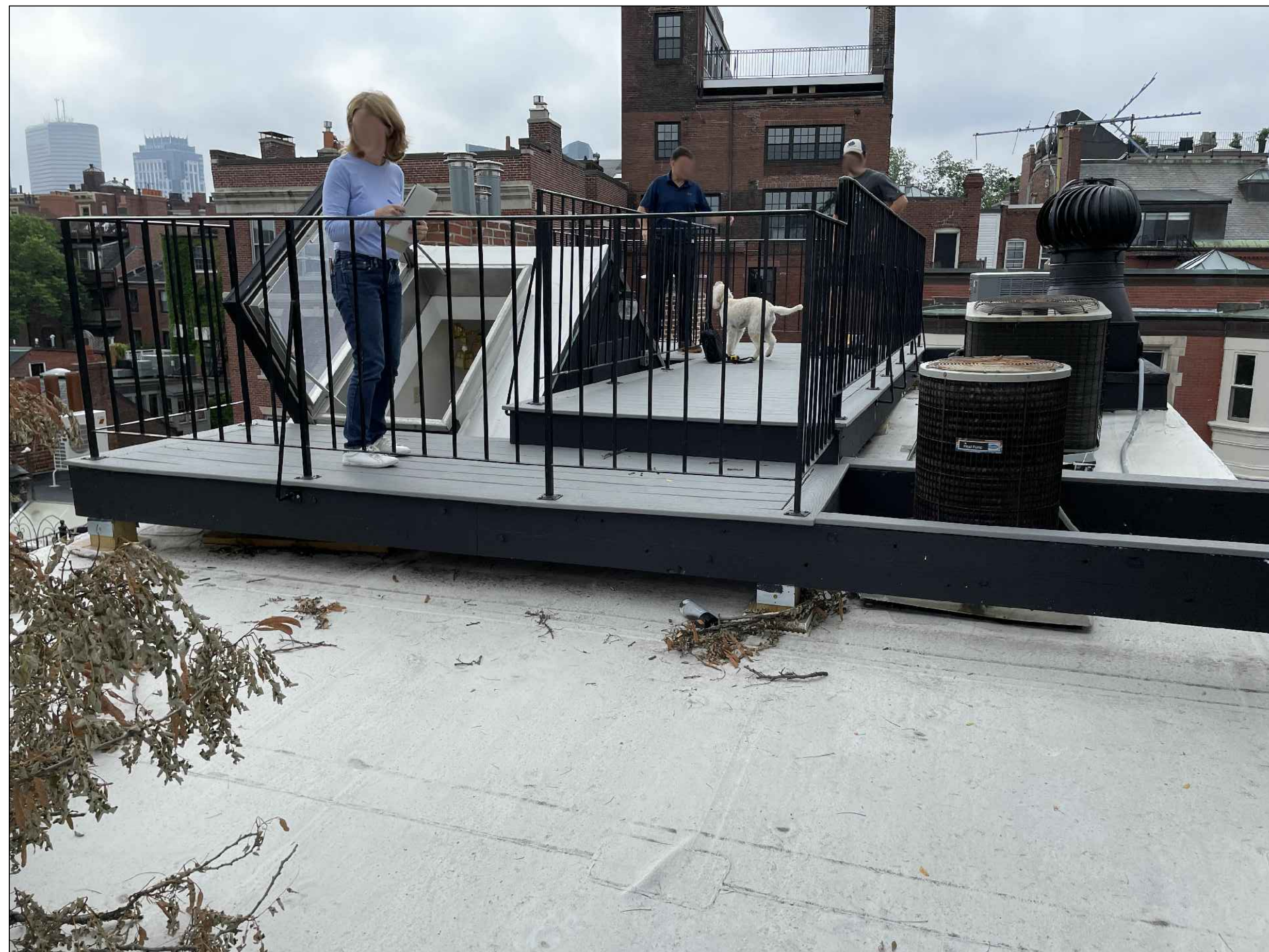
EXISTING ROOF DECK REAR LOOKING SOUTH
