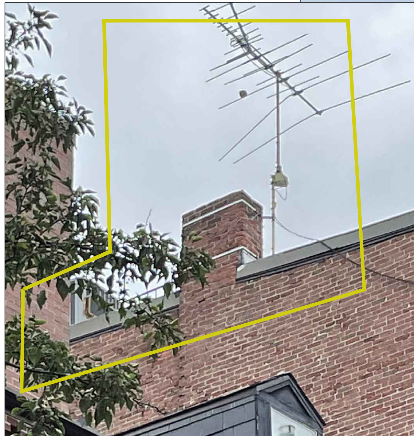
2 CLOSE UP OF VISIBLE ROOF DECK RAILING, ANTENNA, AND CONDENSER UNIT
