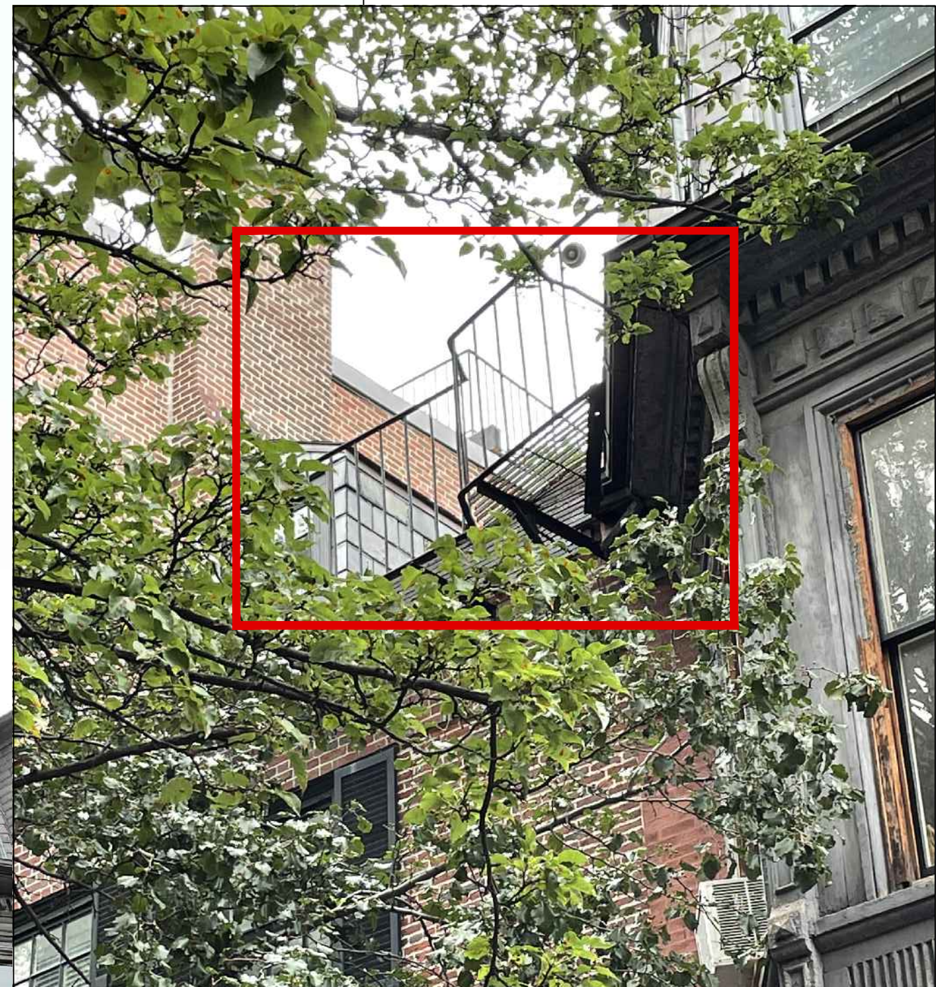
1 CLOSE UP OF VISIBLE ROOF DECK RAILING BEHIND ADJACENT FIRE ESCAPE
