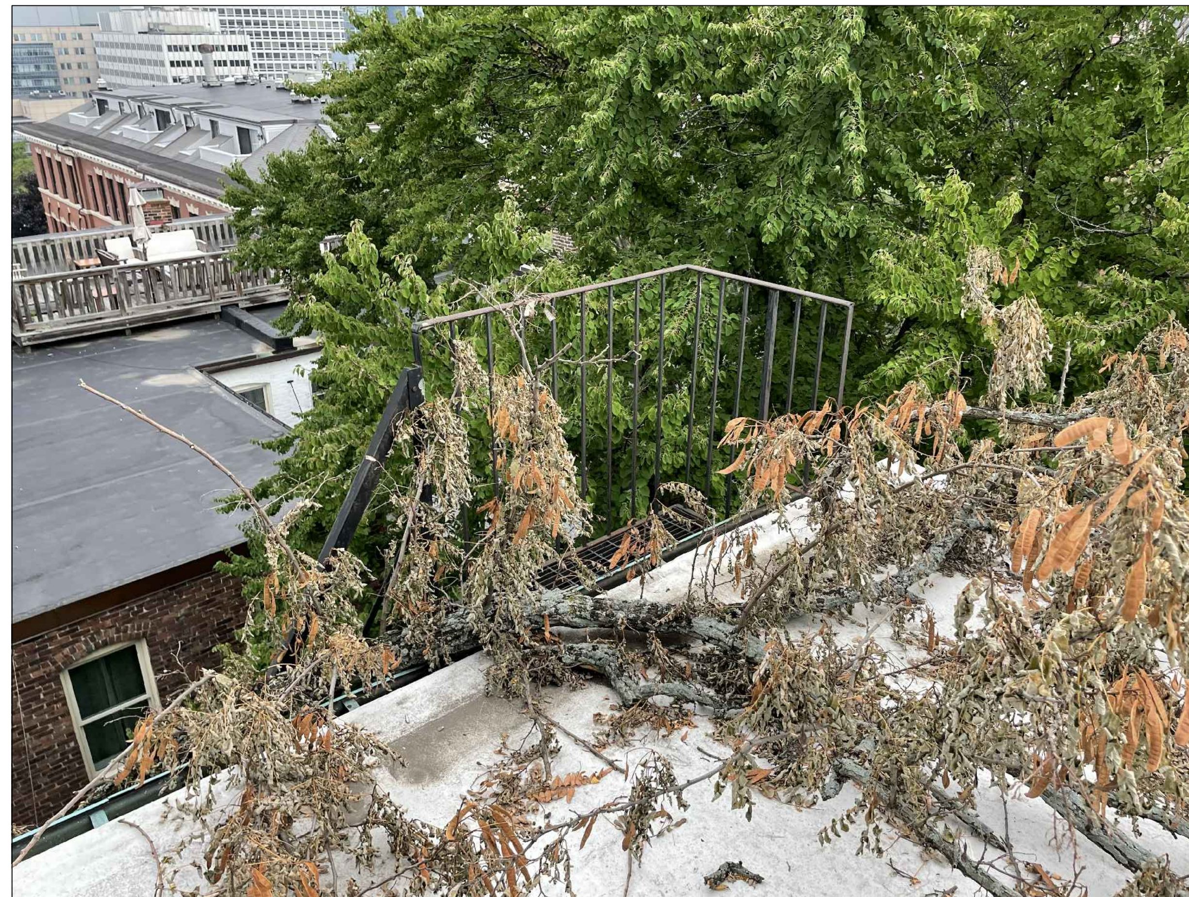
EXISTING REAR FIRE ESCAPE ACCESS
