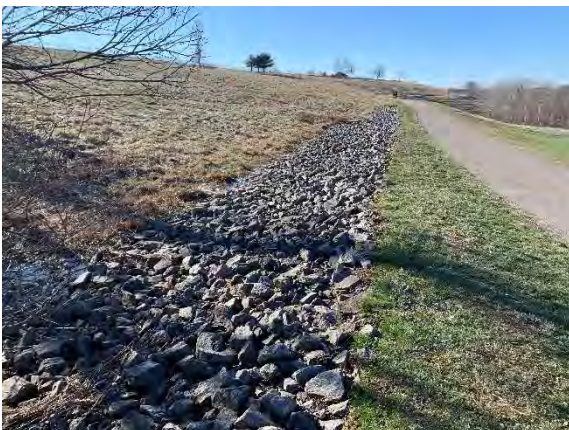
Photograph #13 Drainage swale on northern mid slope.
