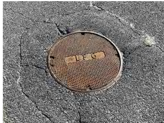
Photograph #16 Manhole cover over landfill system well vault.
