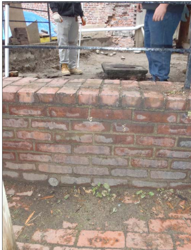
Photograph 4-17. Block drainage pipe likely associated with Feature 13, Upper Patio, view west.
