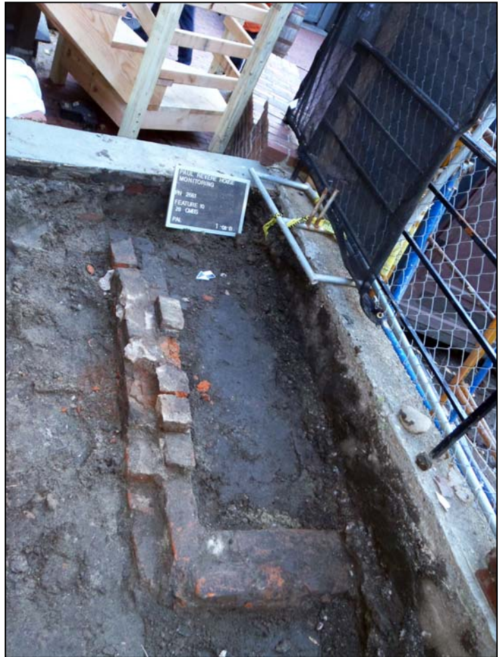
Photograph 4-13. Brick structural element associated with former Angelo Buildings (Feature 10), Upper Patio, view east.
