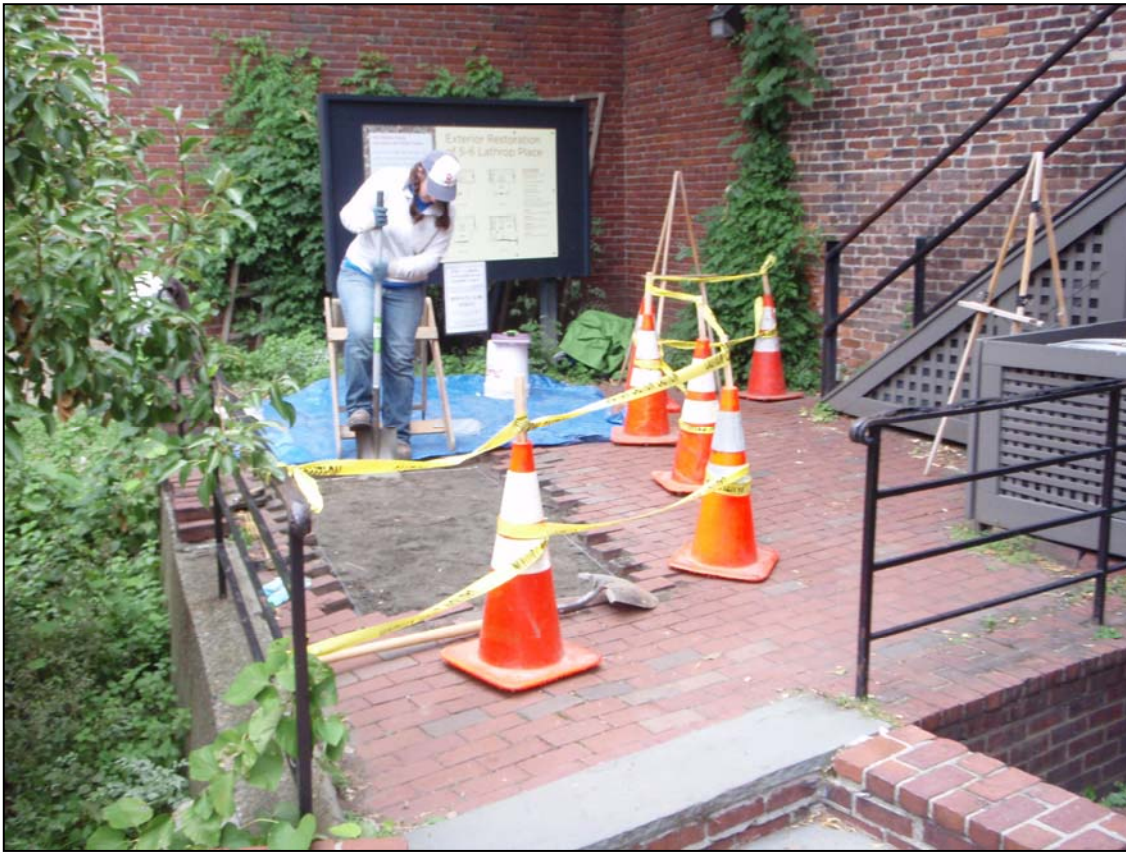
Photograph 4-2. Overview of EU-10 and EU-11, view west.
