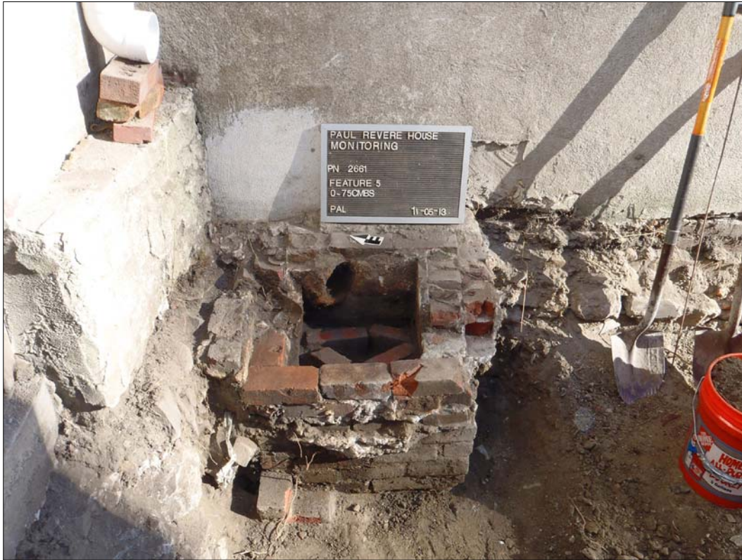
Photograph 4-23. Brick catch basin (Feature 5), Shared Courtyard, view north.
