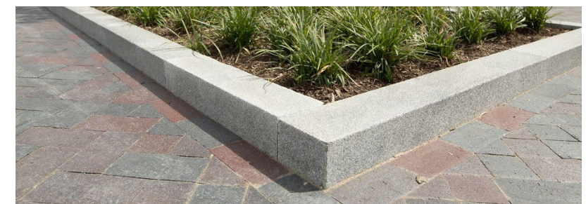
LOW GRANITE CURBING AROUND TREE PLANTING
