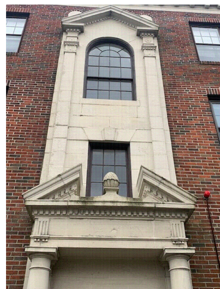
B. 1992 Entry Keystone Repair
