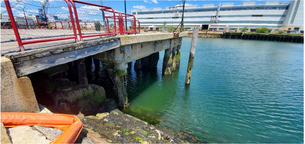
Photo 1: Overall view of the eastern side to Pier 10.
