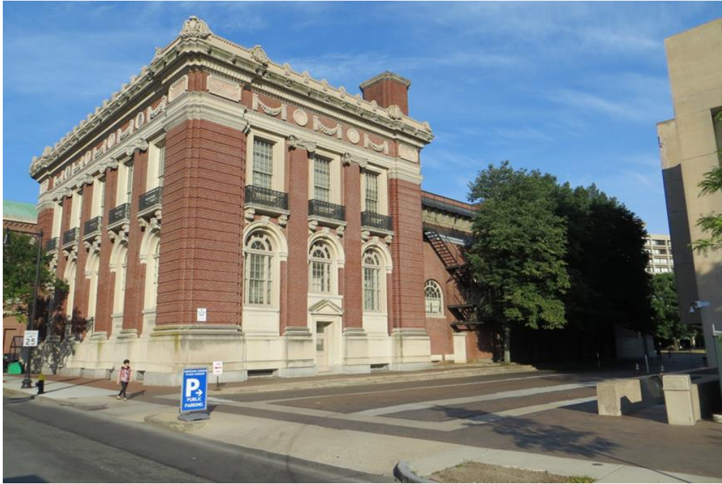
Figure #3. South (facing Huntington Avenue) and east (facing Christian Science Center complex) facades of Horticultural Hall (looking northwest). June 2016.
