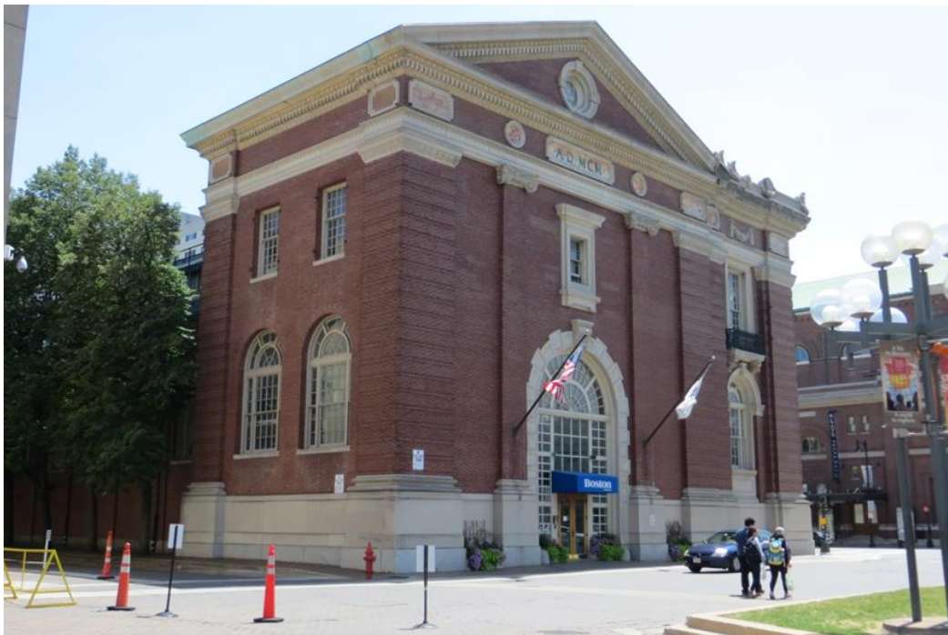
Figure #4. North façade and north end of east elevation (looking southwest). July 2016.
