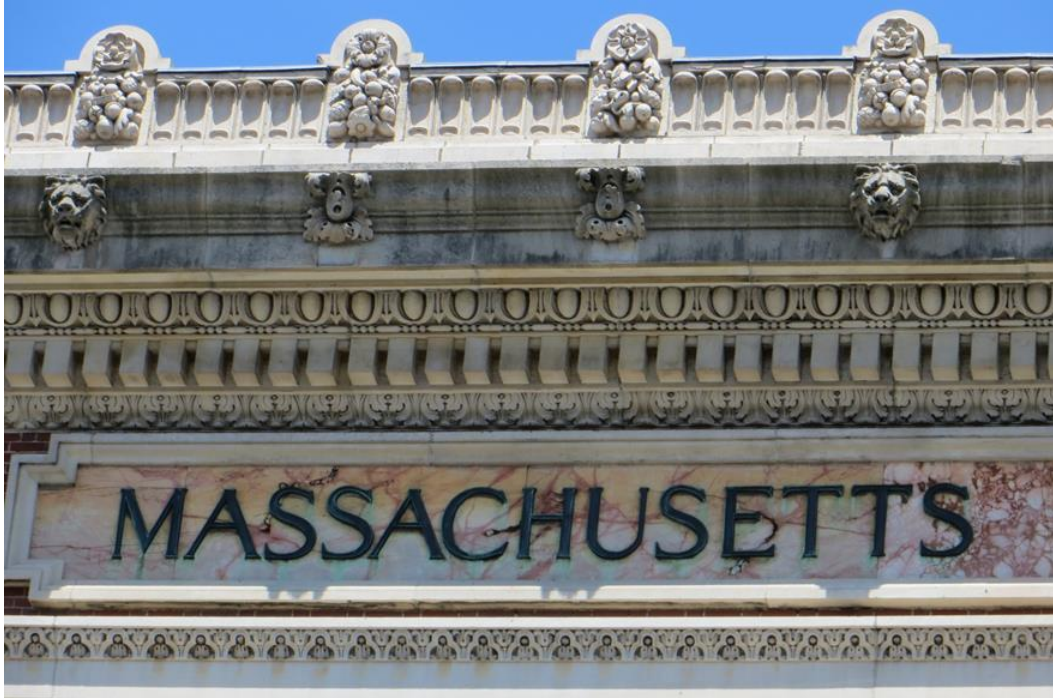
Figure #7. Detail of Cheneau and cornice on west façade (looking east). July 2016.
