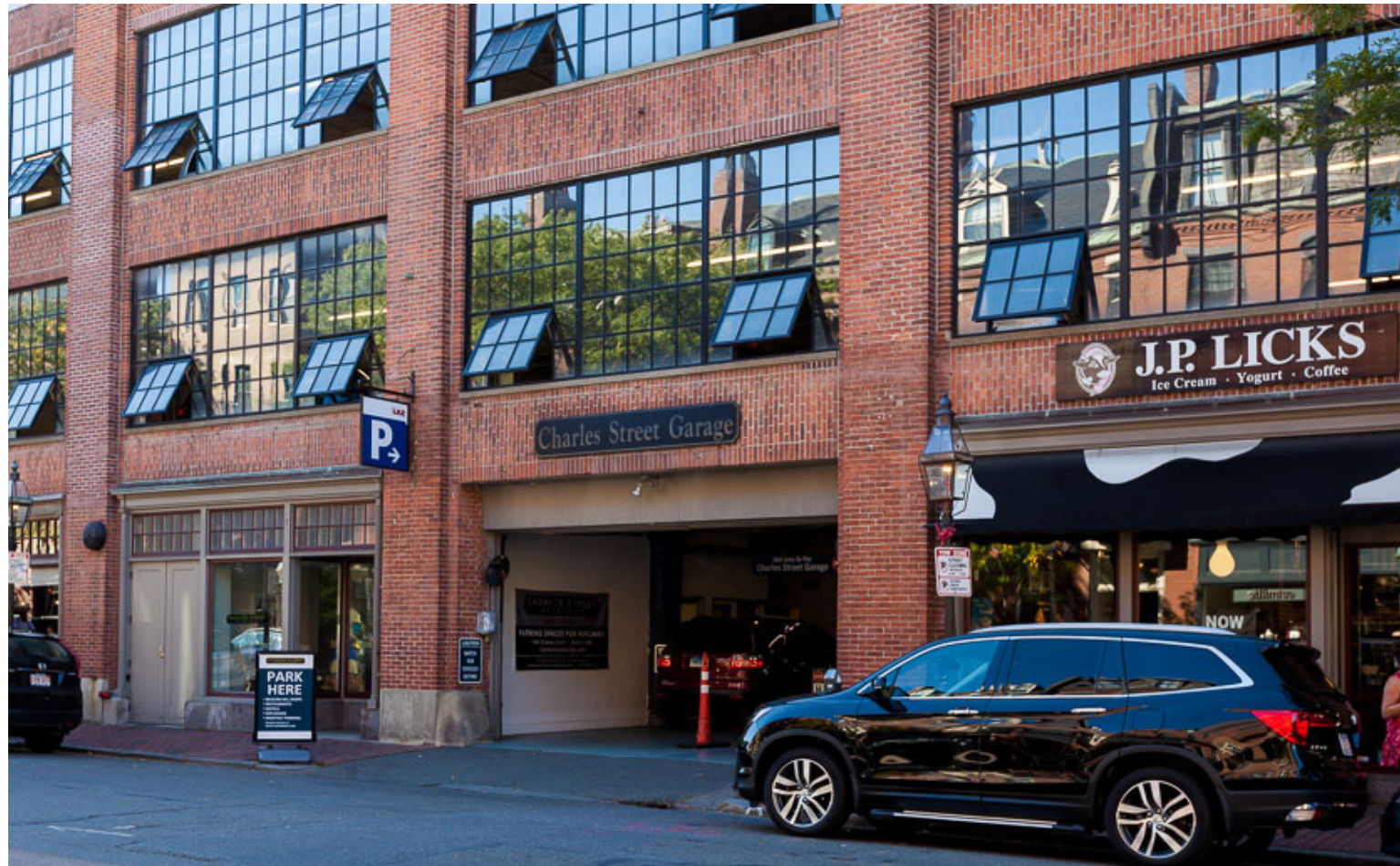
View from Charles Street towards parking entry
