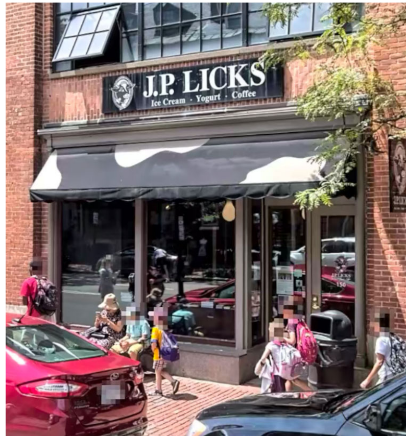
EXISTING VIEW OF RETAIL STOREFRONT
