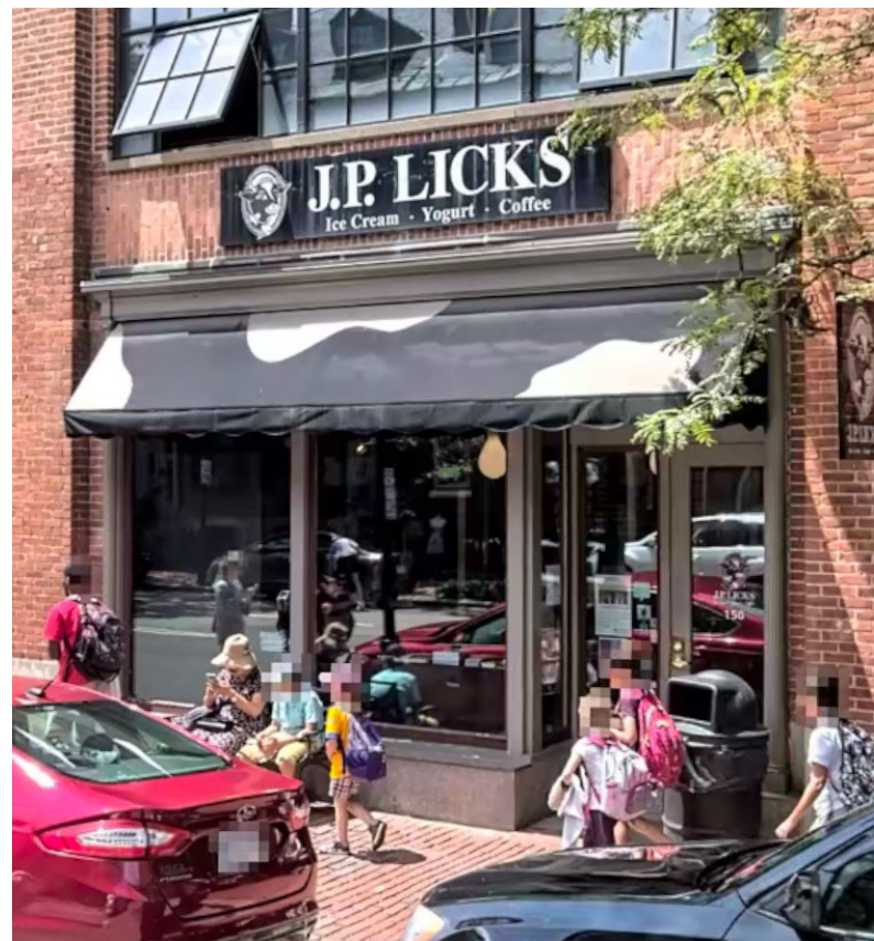
EXISTING VIEW OF RETAIL STOREFRONT
