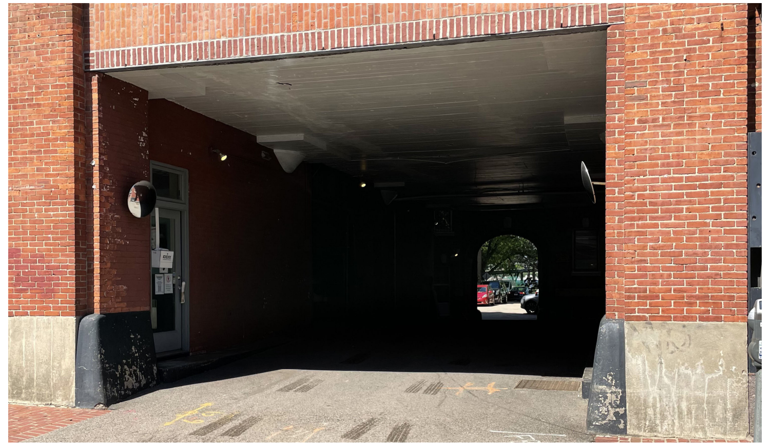
EXISTING VIEW LOOKING WEST
