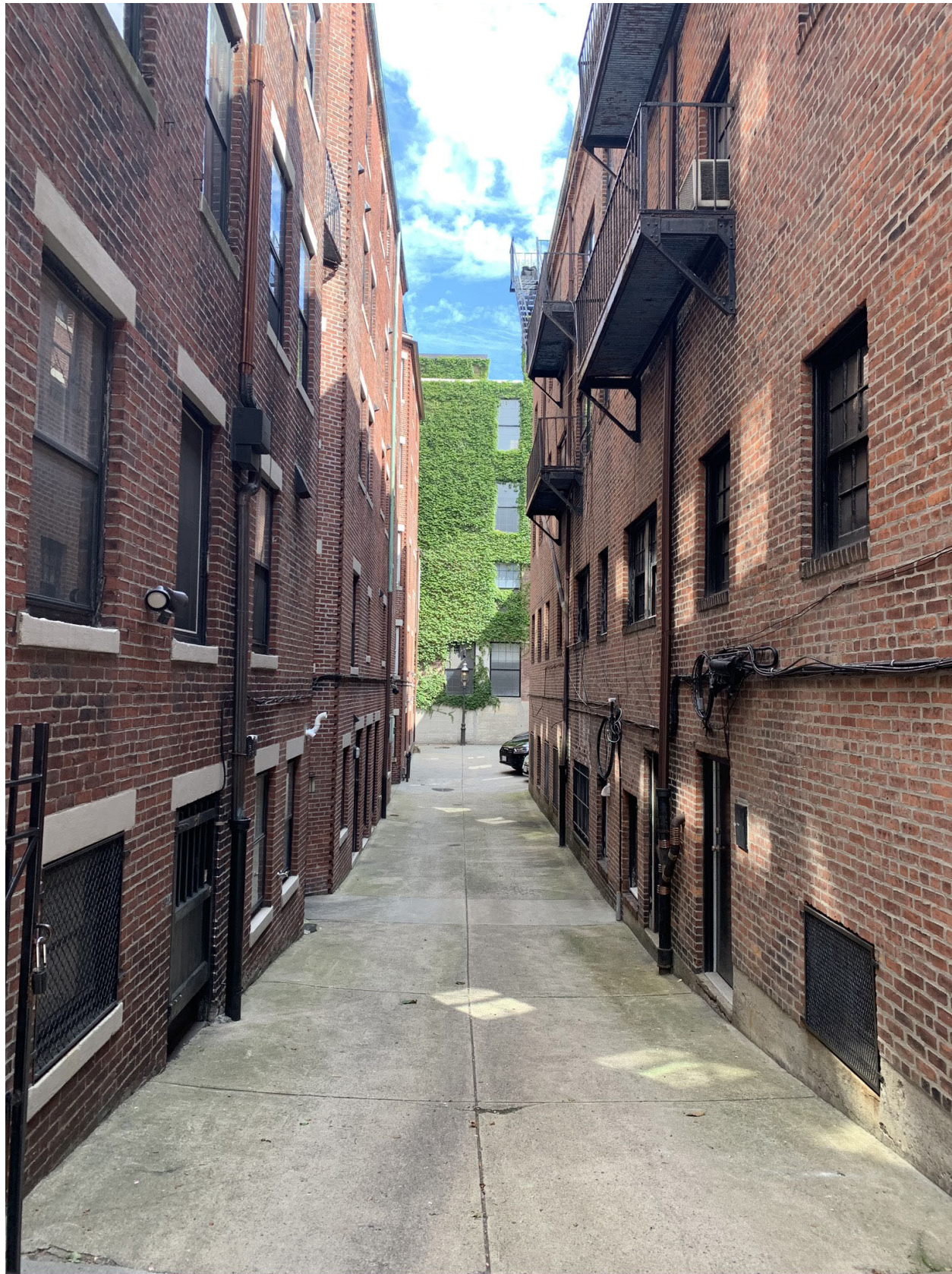
View from Revere Street looking north
