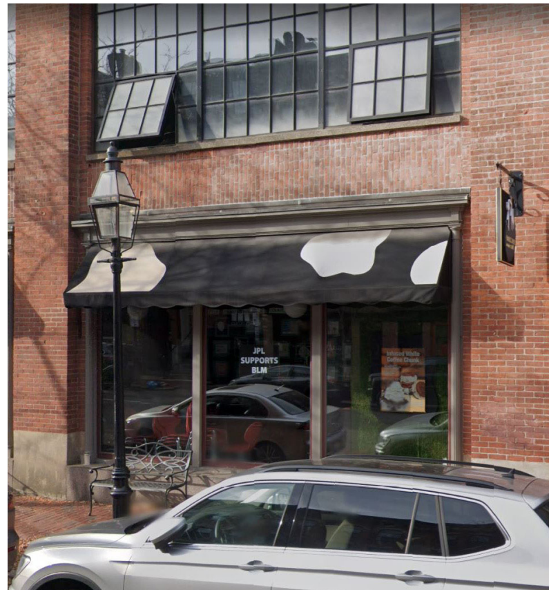
EXISTING VIEW OF RETAIL STOREFRONT
