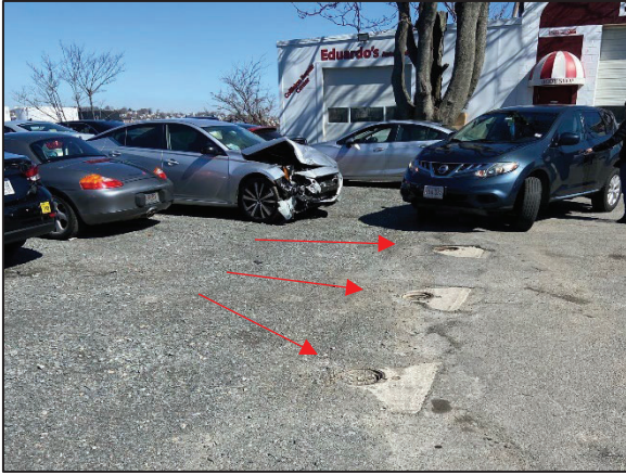
Photo 1 Overview of the abandoned gasoline UST fill ports, as indicated by the red arrows.
