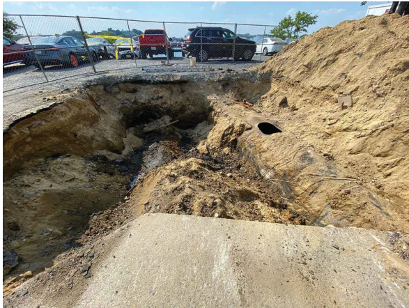
Photo 5: Excavation of Gasoline USTs.
