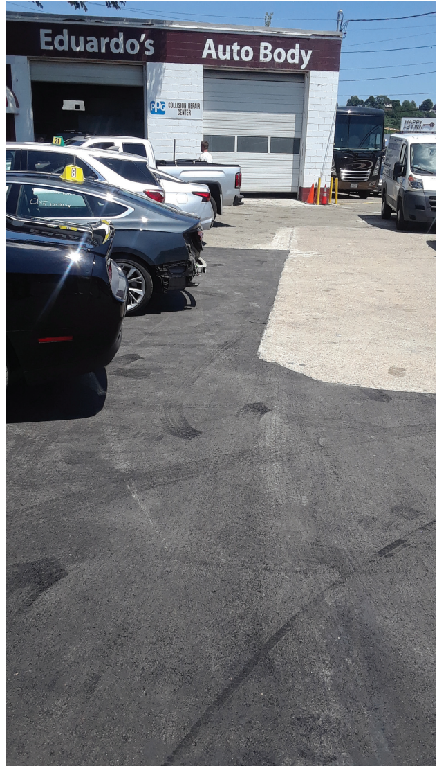
Photo 8: Final Paving looking north.
