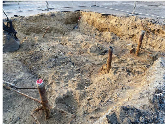
Photo 4: Excavation of Gasoline USTs.
