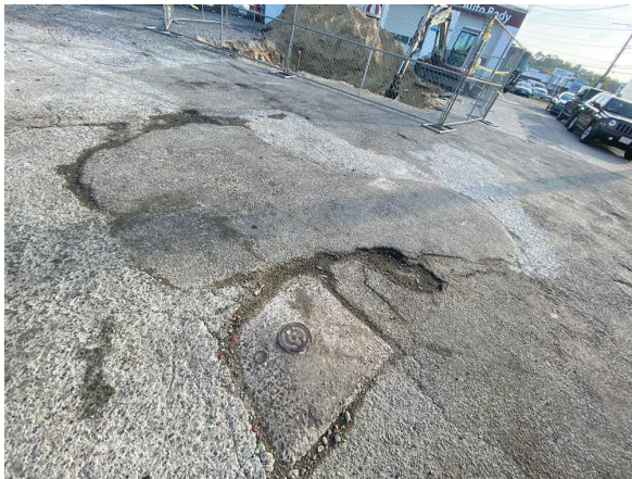
Photo 3: Excavation of Gasoline USTs.
