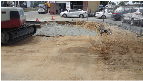
Photo 6: Backfill of Gasoline USTs.
