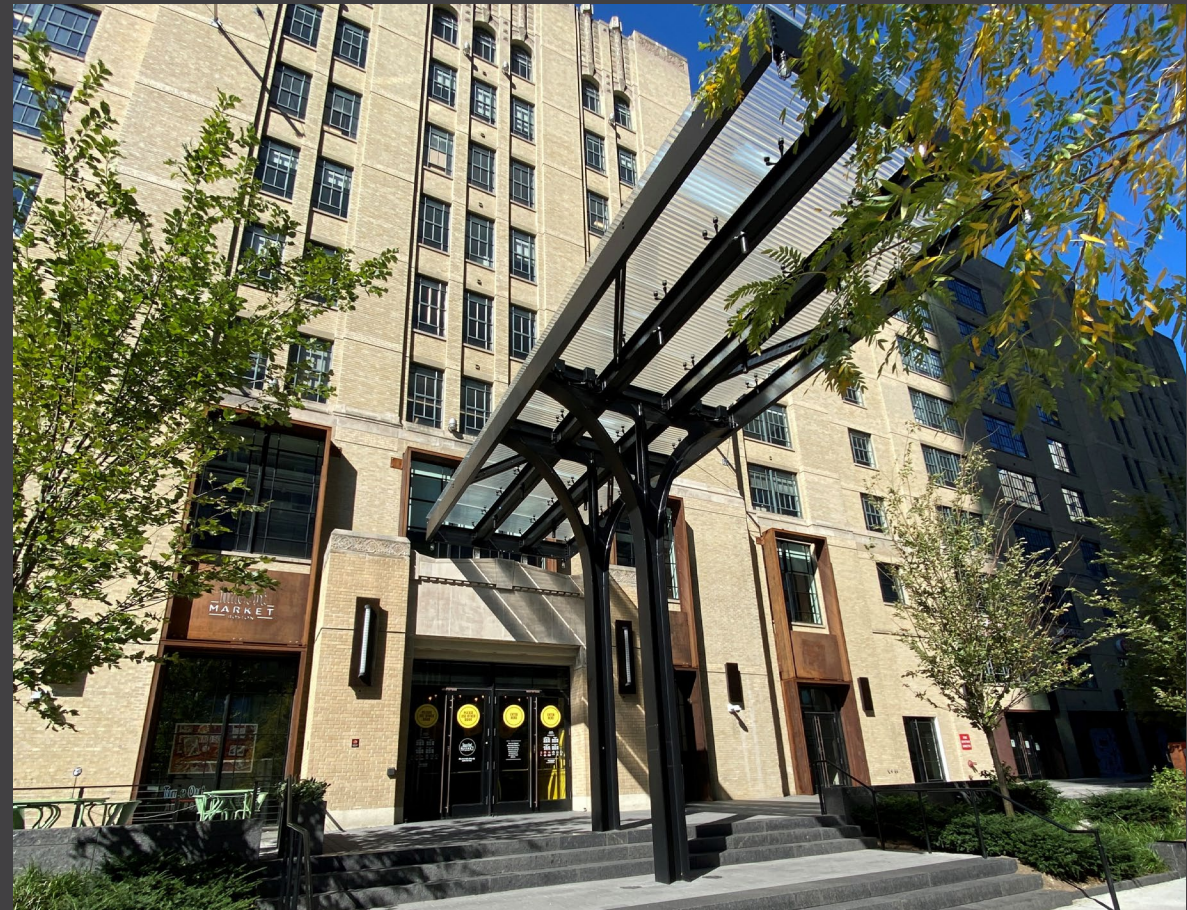
401 Park Brookline Avenue Canopy
