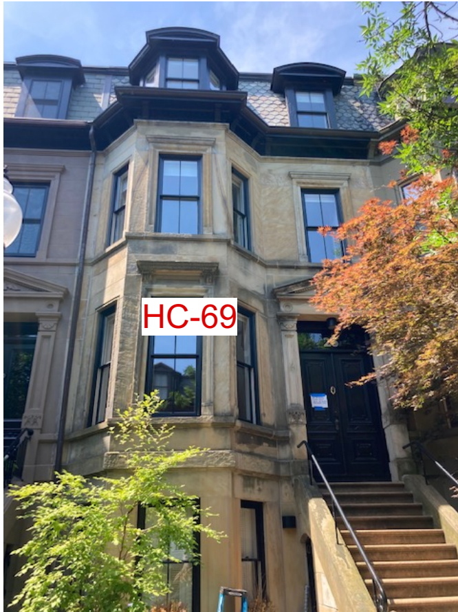
#26 HOLYOKE STREET EXISTING FACADE CONDITION.
