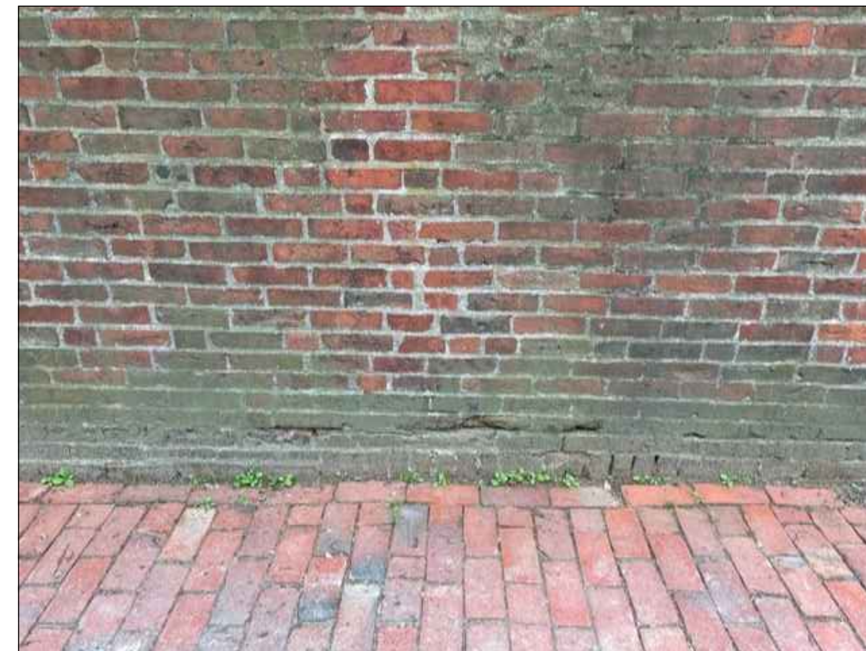
CONDITION OF MASONRY WALL
