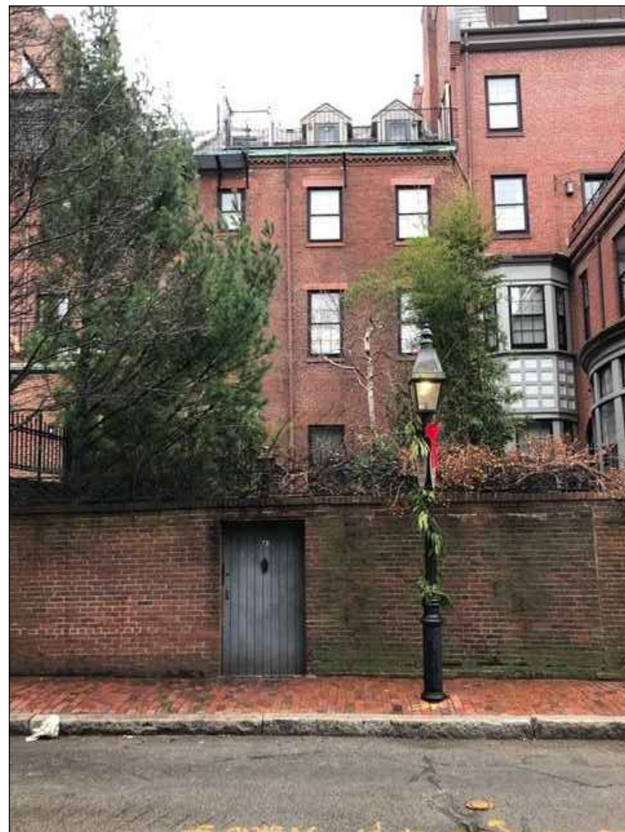
73 BEACON STREET REAR ELEVATION
