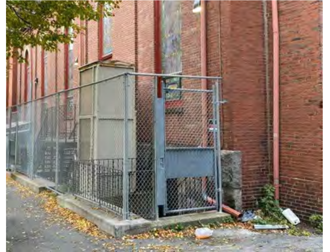
EXTERIOR LIFT TO LEVEL 1
