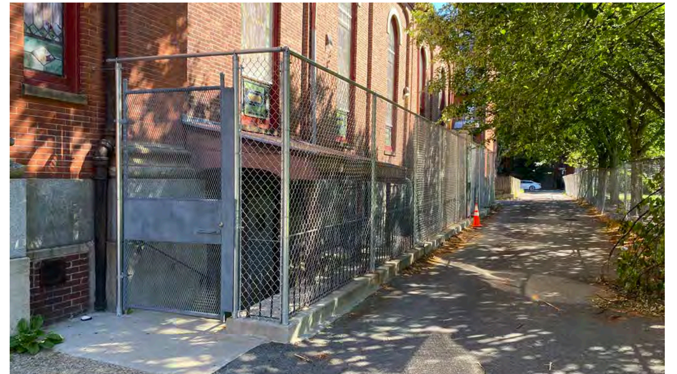
CHAIN LINK FENCE
