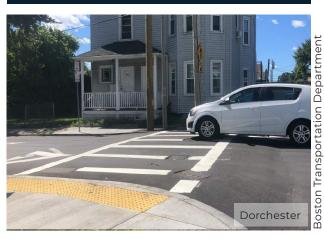
A crosswalk that stays level with the sidewalk. Similar to a speed hump, vehicles must ramp up to a raised crosswalk, thereby reducing driving speeds and increasing comfort for people walking.
