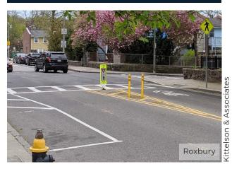
A quick-build median uses paint and flex posts to form a median between two-way traffic. Medians help to slow driving speeds at intersections and draw attention to crosswalks.
