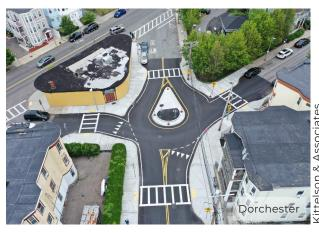
A small roundabout with a mountable central island that aids in directing vehicle traffic, slowing driving speeds, and facilitating safe pedestrian crossings.
