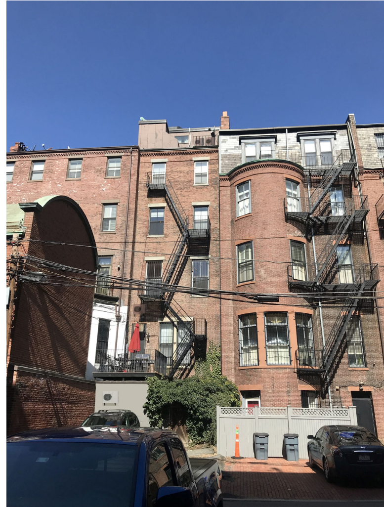
2 UNITS ON THE ROOF, 1 UNIT ON THE BACK WALL (BRICK), 1 UNIT ON THE LOWER BACK WALL.
