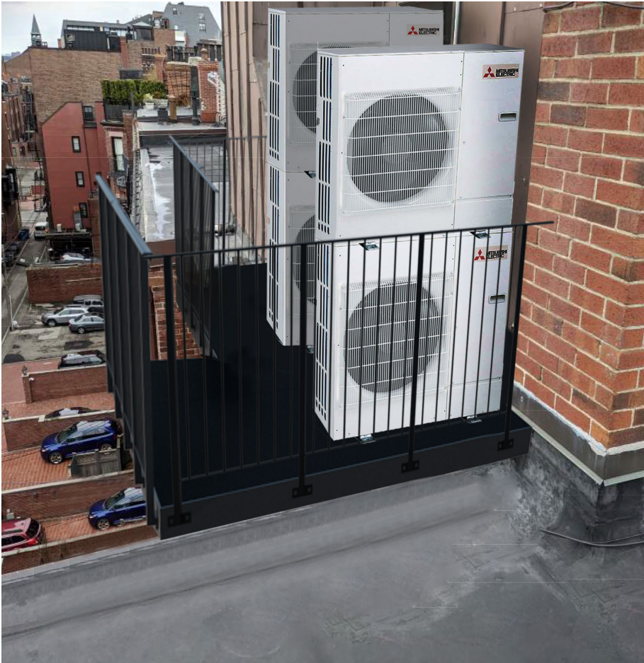
PREVIOUSLY PROPOSED HVAC UNITS WITH GUARD RAILINGS
