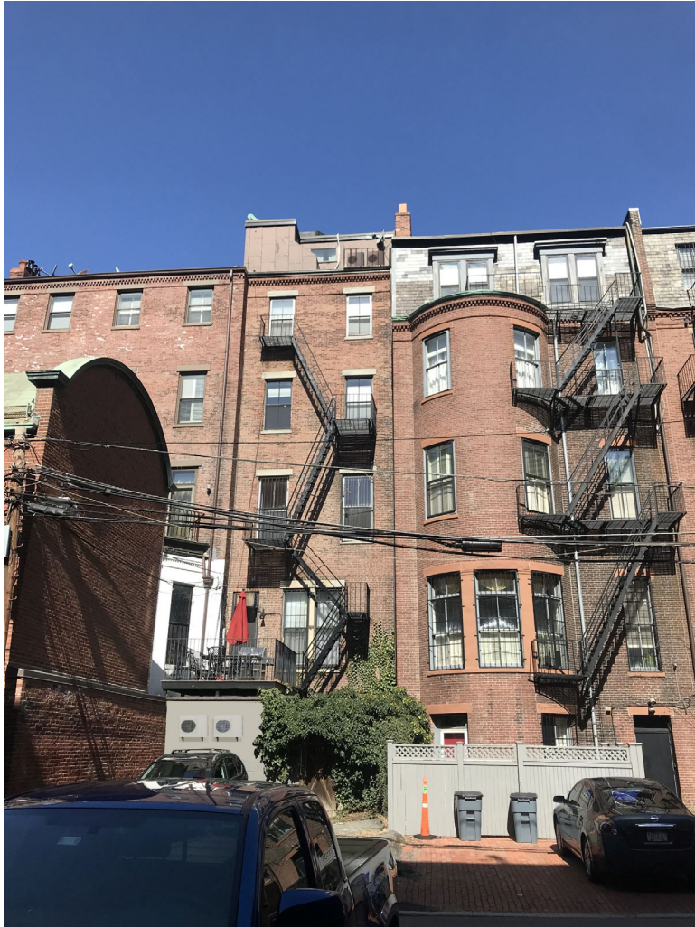
2 UNITS ON THE ROOF, 2 UNITS ON THE BACK WALL
