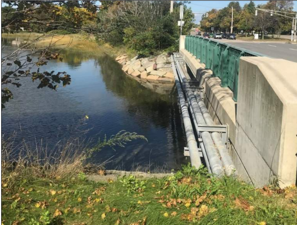
Photo 5 – Patten’s Cove culvert crossing facing northwest. (10/10/18)
