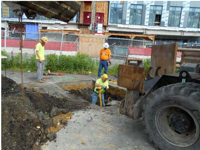
Photo 7: Backfilling/compacting within HA19-TP2
