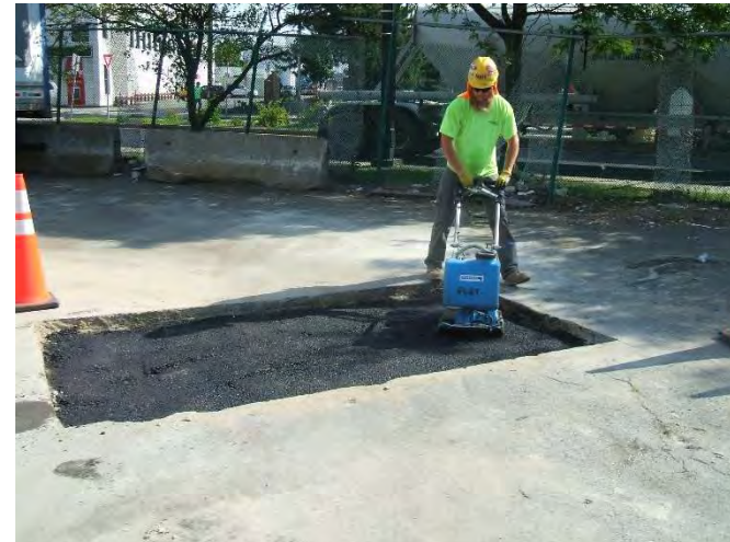
Photo 23: Completed/backfilled test pit at HA19-TP6
