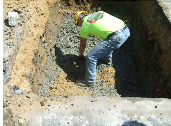
Photo 18: Hand excavation to expose top of tunnel at HA19-TP5
