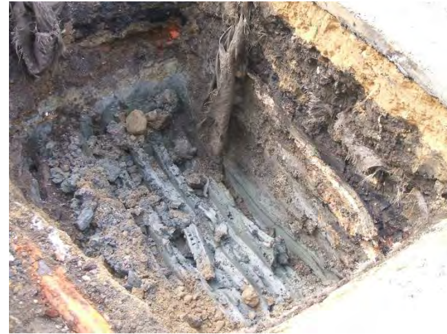
Photo 6: Clay (hydraulic fill) material encountered at depth of approx. 5 ft below existing site grades at HA19-TP2
