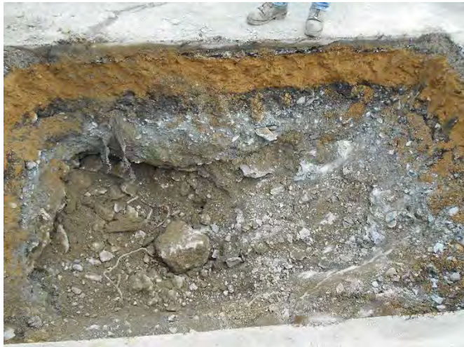
Photo 26: View looking into HA19-TP7 excavation
