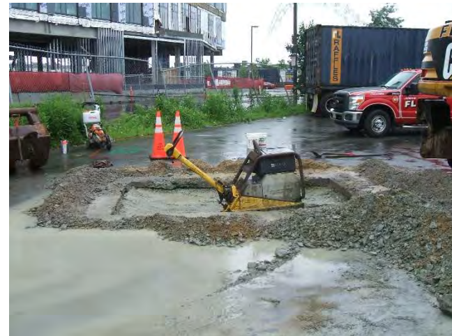
Photo 12: Backfilling/compacting within completed HA19-TP3 test pit
