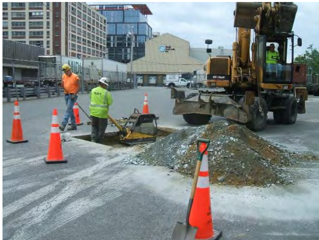
Photo 15: Backfilling/compacting within completed HA19-TP4 test pit
