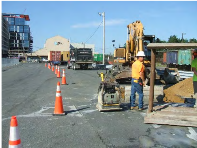
Photo 28: View looking east at HA19-TP8 excavation
