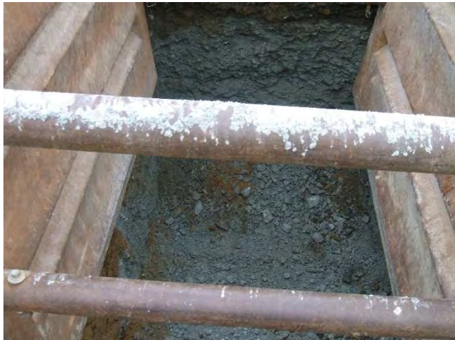
Photo 30: Trench box installed for temporary excavation support at HA19-TP8
