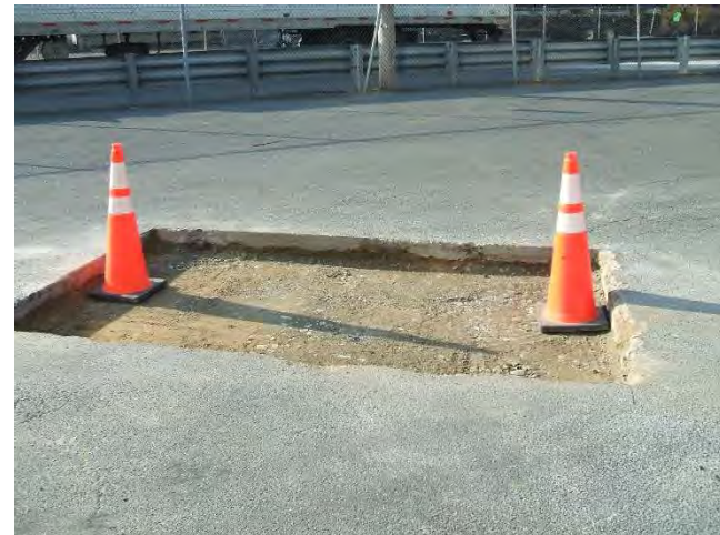
Photo 16: Completed/backfilled test pit at HA19-TP4
