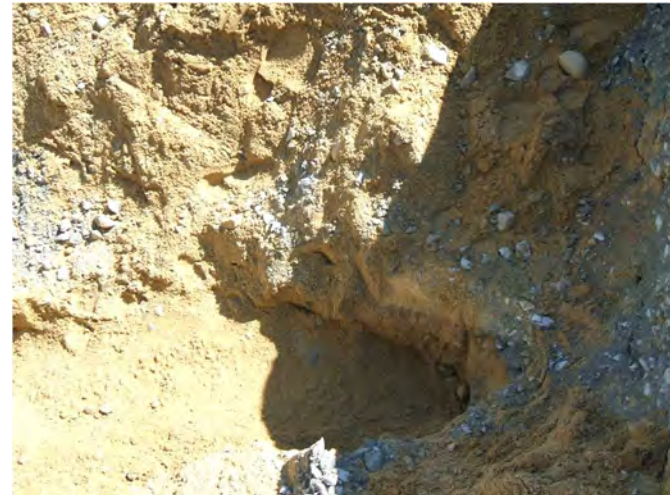
Photos 34 and 35: Hand excavated to top of tunnel protective slab at depth of 6.5 to 6.9 ft below existing site grades at HA19-TP9
