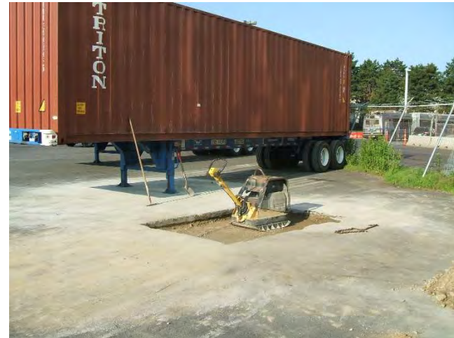
Photo 4: Backfilled/compacted test pit at HA19-TP1
