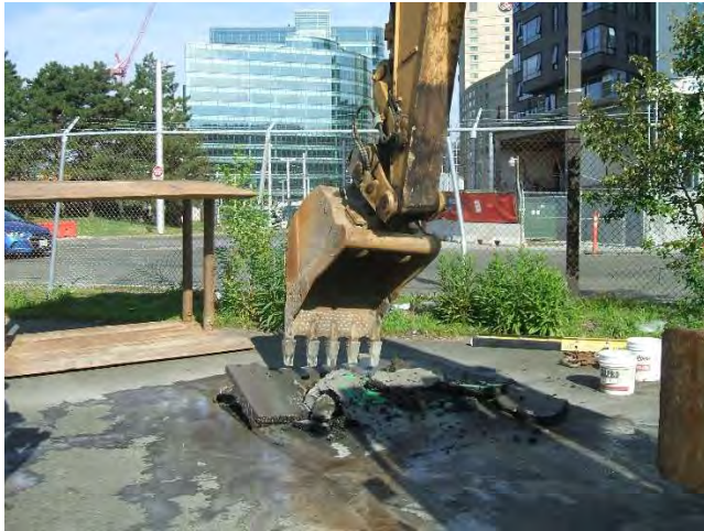
Photo 1: View looking west at HA19-TP1
