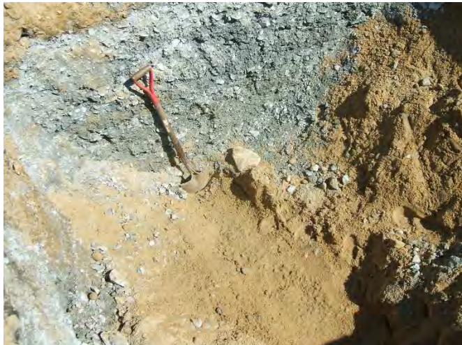
Photos 34 and 35: Hand excavated to top of tunnel protective slab at depth of 6.5 to 6.9 ft below existing site grades at HA19-TP9
