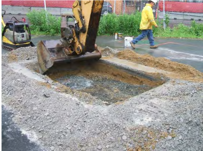
Photo 9: View looking west at HA19-TP3 excavation
