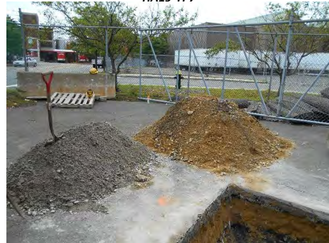
Photo 27: View of excavated material generated from HA19-TP7 excavation
