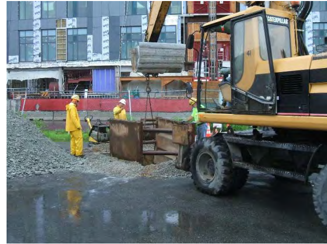
Photo 10: Installing trench box for temporary excavation support at HA19-TP3
