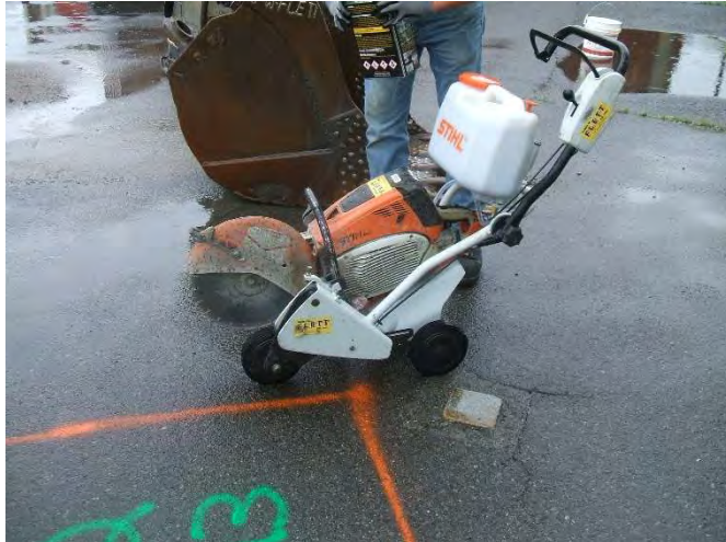
Photo 5: Saw cutting asphalt at HA19-TP2
