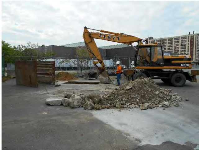
Photo 24: View looking south at location of HA19-TP7
