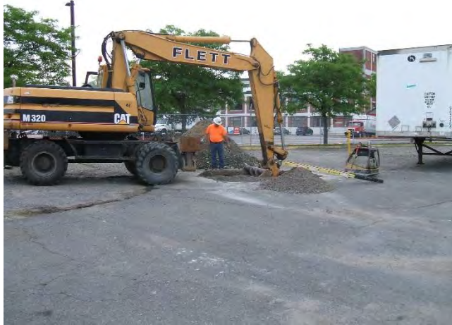
Photo 32: View looking east at HA19-TP9 excavation
