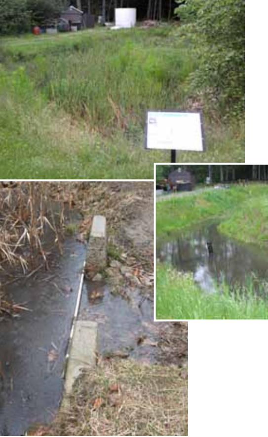
Detention ponds can be effective for many common stormwater pollutants but efforts to reduce operation and maintenance costs should be considered during system design.
