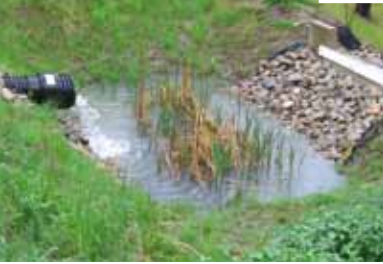
Bioretention systems are the workhorse of LID approaches and offer flexible, adaptive and reliable treatment of stormwater runoff.
