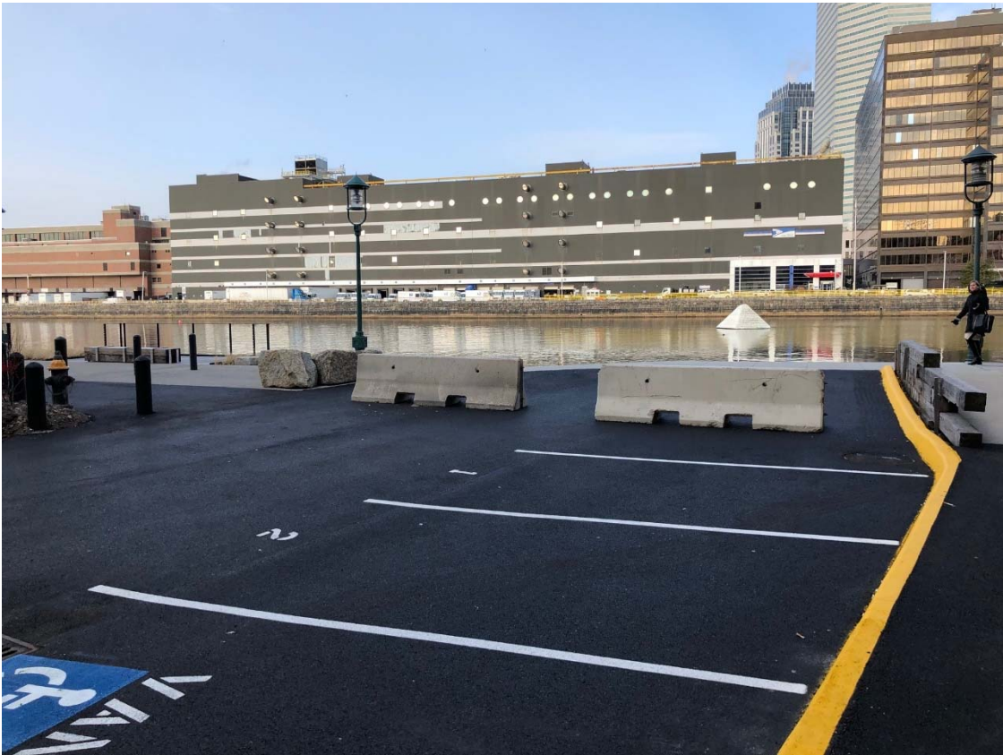
View northwest toward project site from Necco Court
