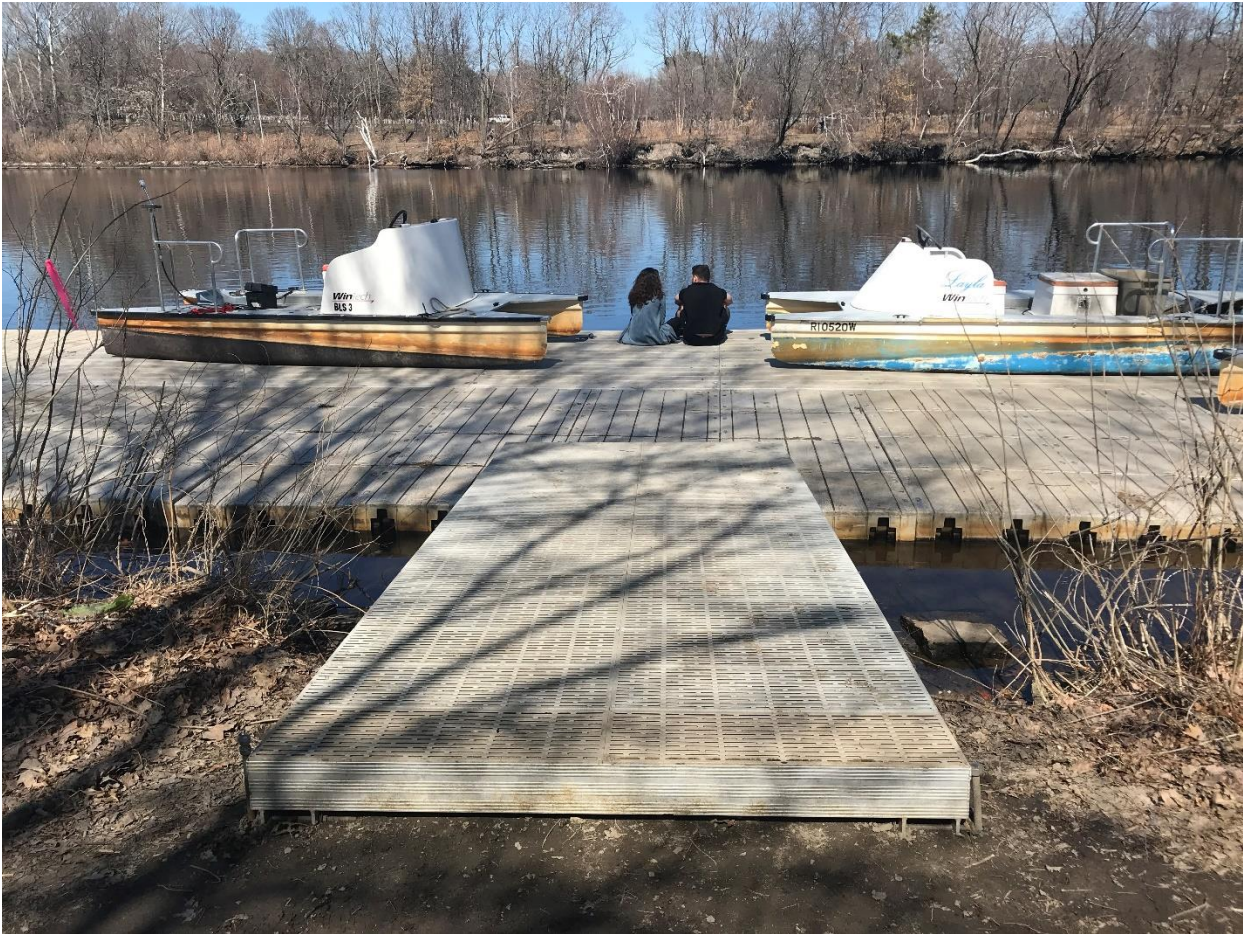
Photo of ramp to temporary dock:
