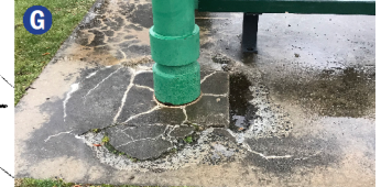
Cracked Concrete
