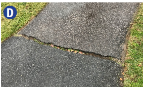
Pathway Cracking
