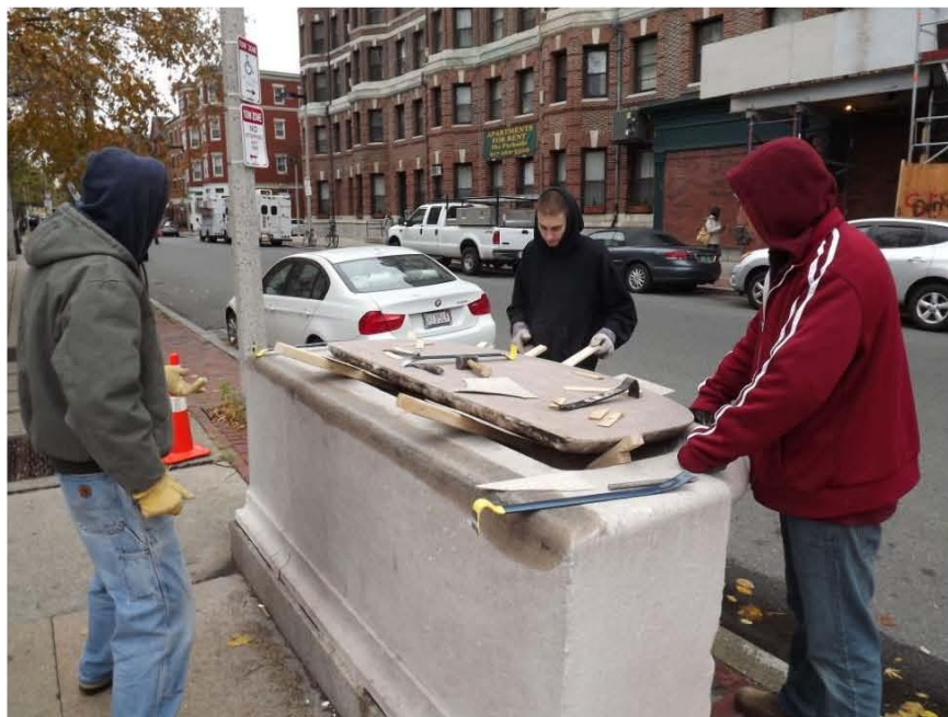
2013: CONSERVATORS REMOVED THE EXISTING GRANITE COVER OF THE HORSE TROUGHS AND RESEALED THE JOINTS.
