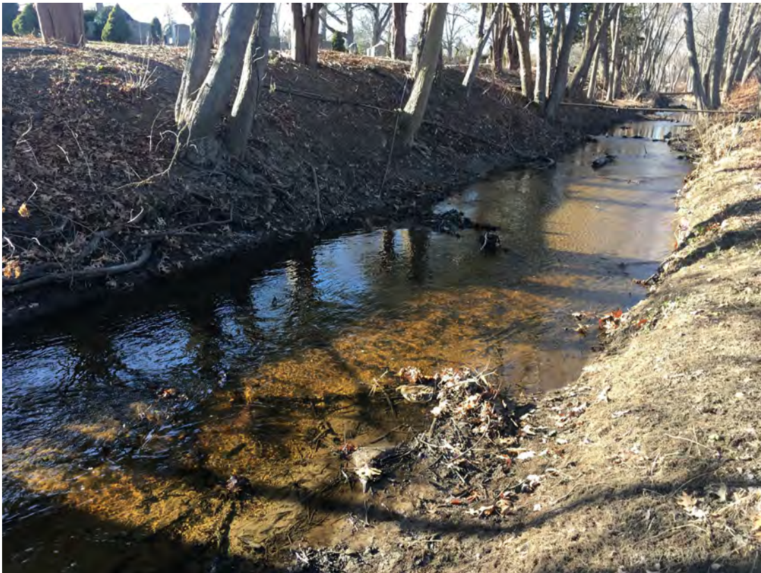
Other Typical Minor Logs, Branches, Debris, Leaf Dams to be Removed
