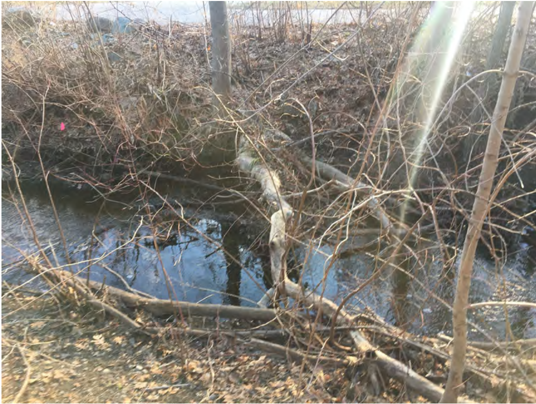
STR9: Logs over Stream and Branches in and over Stream to be Removed
