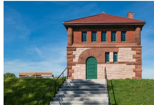
Fisher Hill Reservoir Gatehouse
