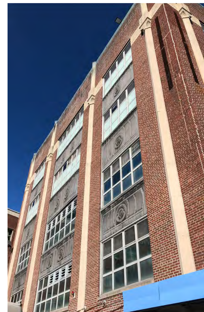
South West Entry Detail
