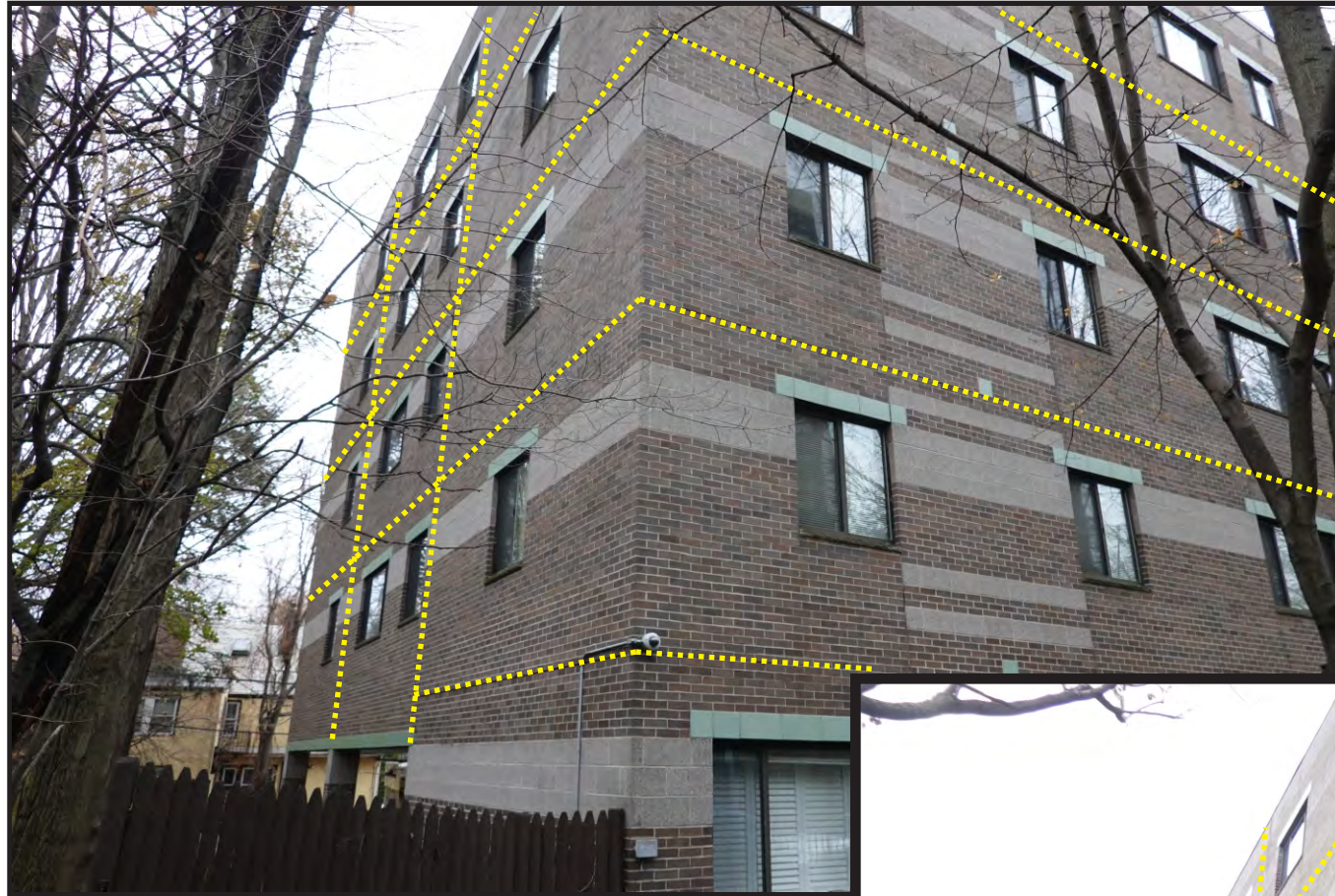
APPROXIMATE LOCATIONS OF EXPANSION JOINTS
