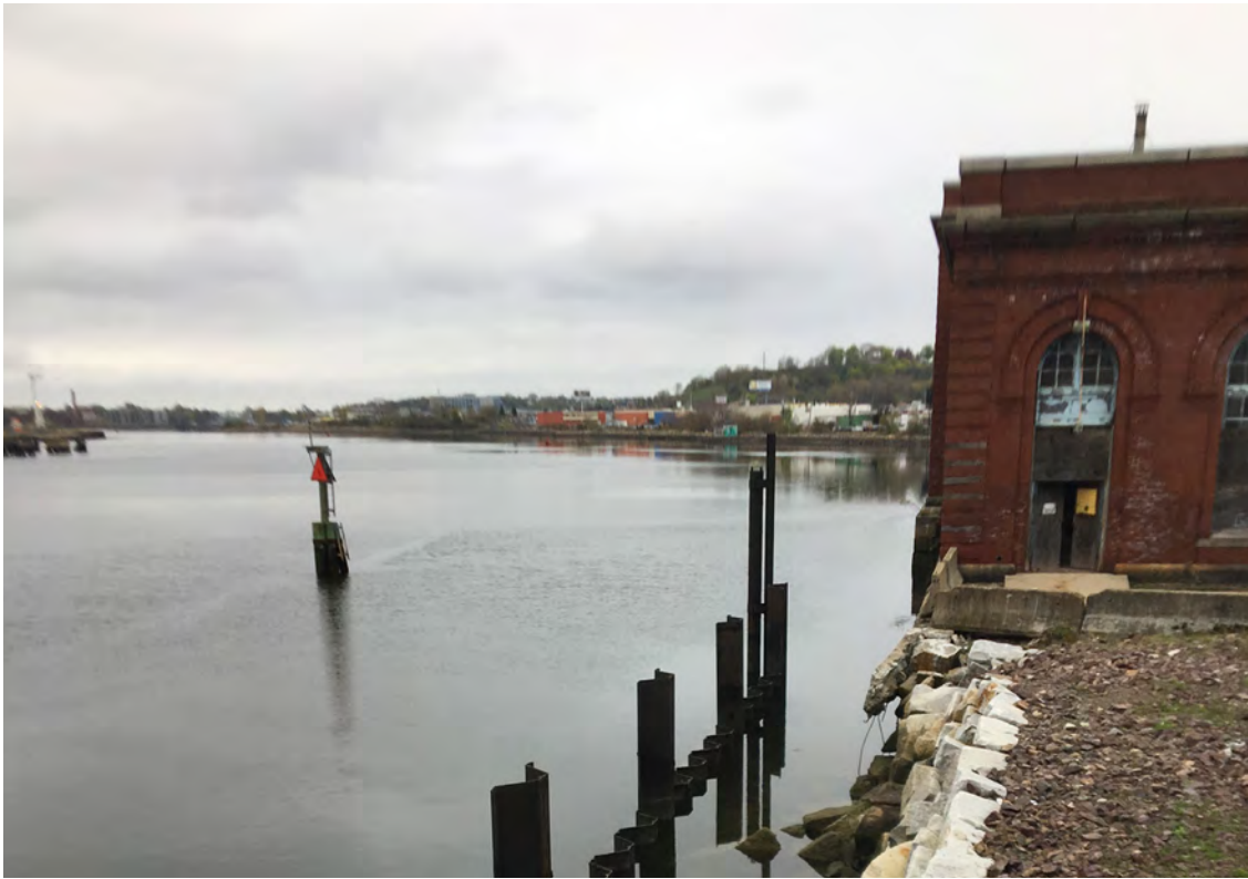
Southwestern corner of the building and Chelsea Creek
