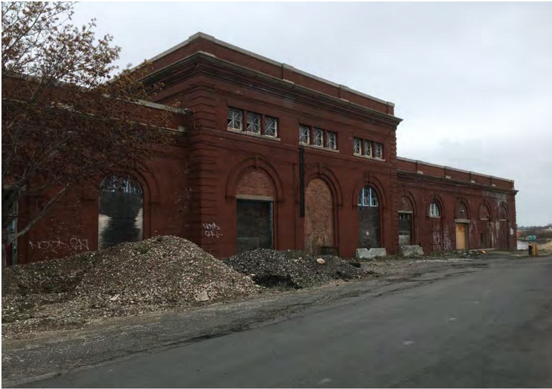
Southern face of the building
