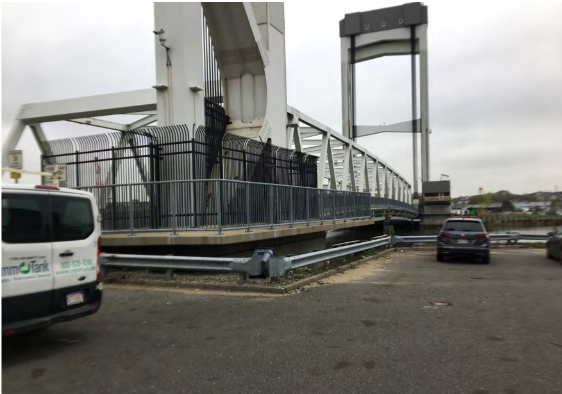
Chelsea Street bridge easement area
