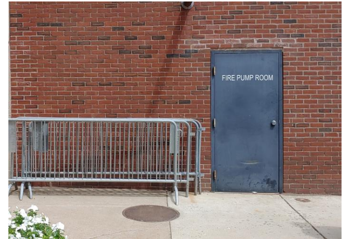
Garage Entrance & Access Door To Be Protected
