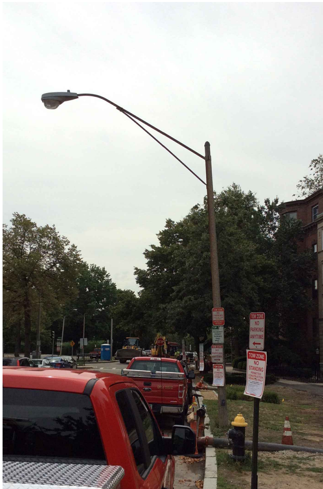
EXISTING PHOTOGRAPHIC VIEW 42.343889°, -71.094967°
