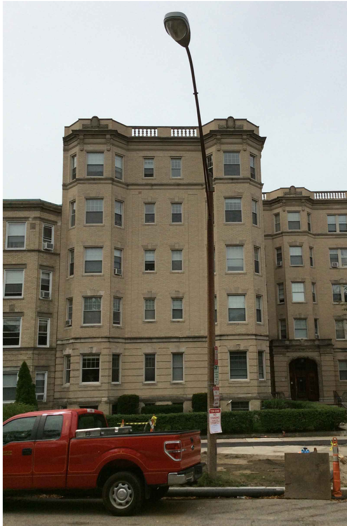
EXISTING PHOTOGRAPHIC VIEW 42.343889°, -71.094967°
