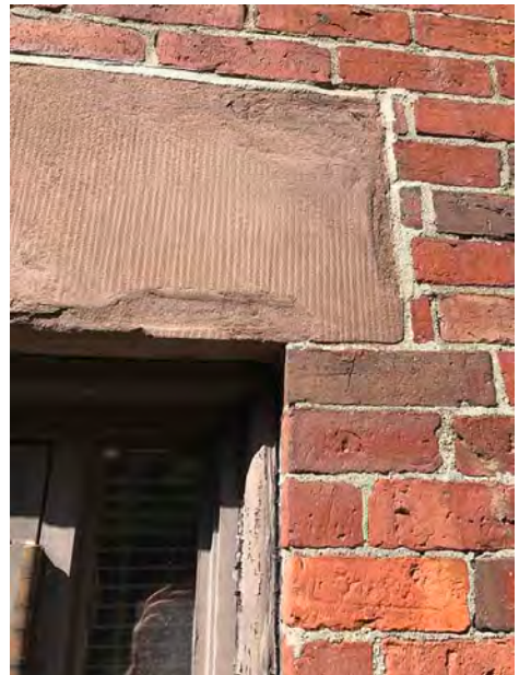
RESTORE MISSING SURFACE WITH MATCHING REPAIR MORTAR
