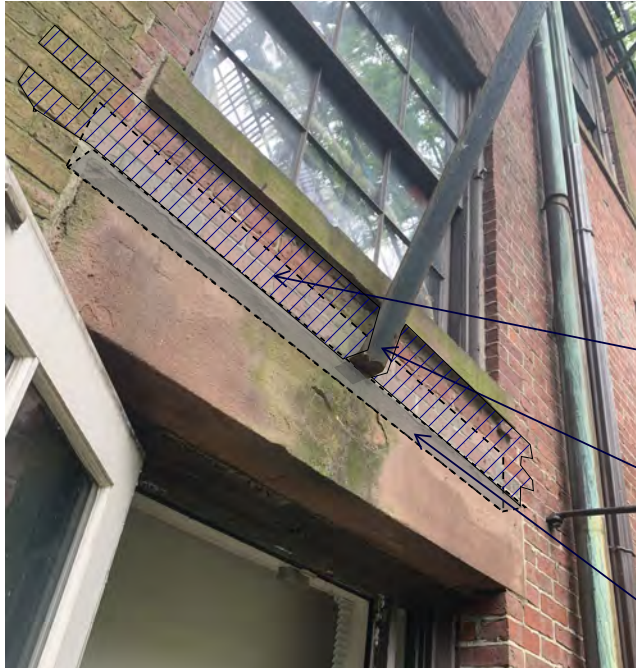
EXISTING FIRE ESCAPE BRACKET BETWEEN BROWNSTONE LINTEL & SILL EMBEDDED IN BRICKWORK
