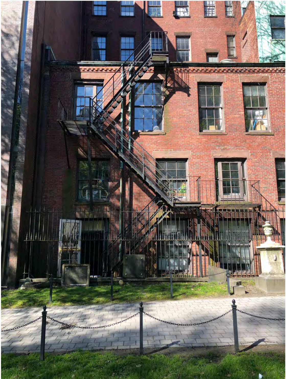
REAR FACADE OF 2 PARK STREET FROM GRANARY BURYING GROUND
