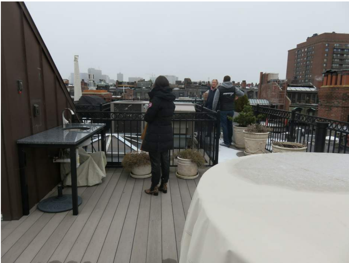
EXISTING ROOF DECK - SKYLIGHT
