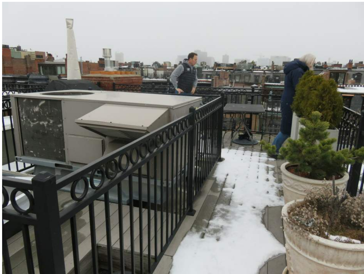
EXISTING ROOF DECK - MECHANICAL
