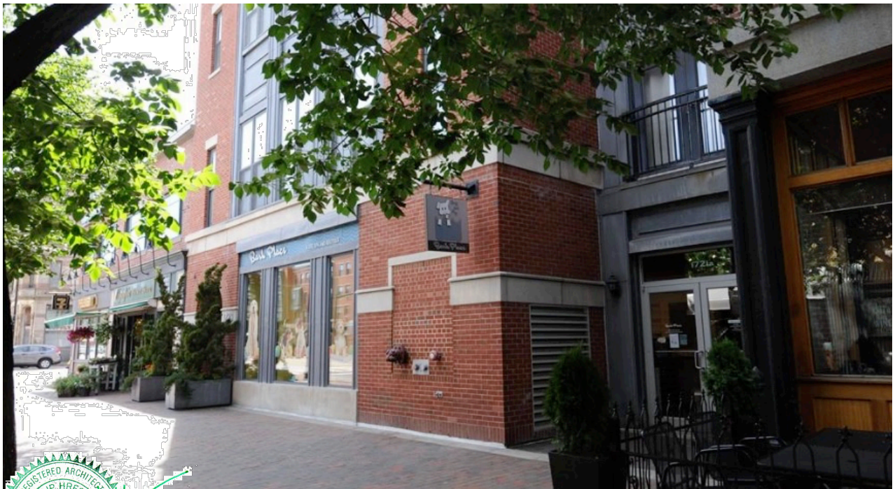
PHOTO 2 -EXISTING FRONT ELEVATION STREET VIEW
