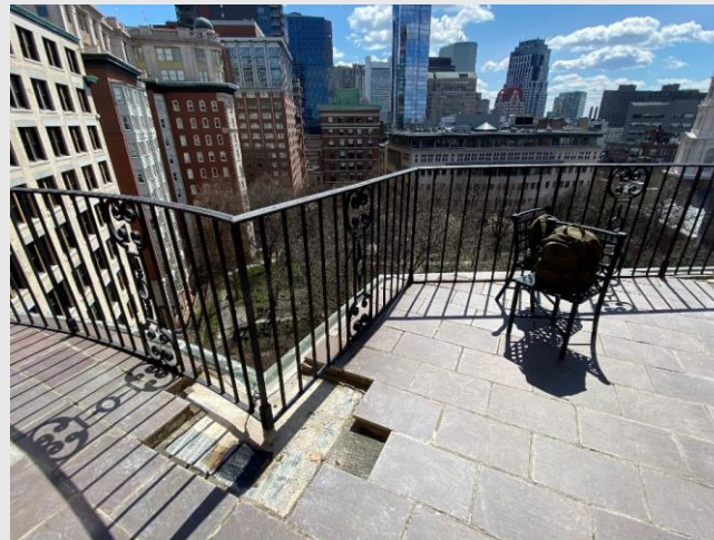
Overview of Fifth-floor balcony
