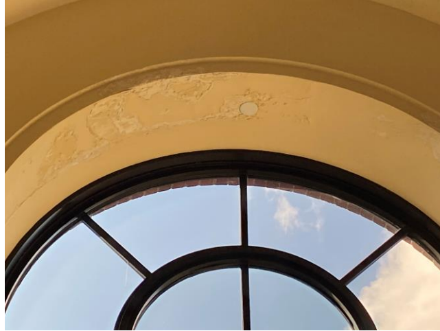
Photo 6: Damaged interior water damage below fifth-floor balcony.
