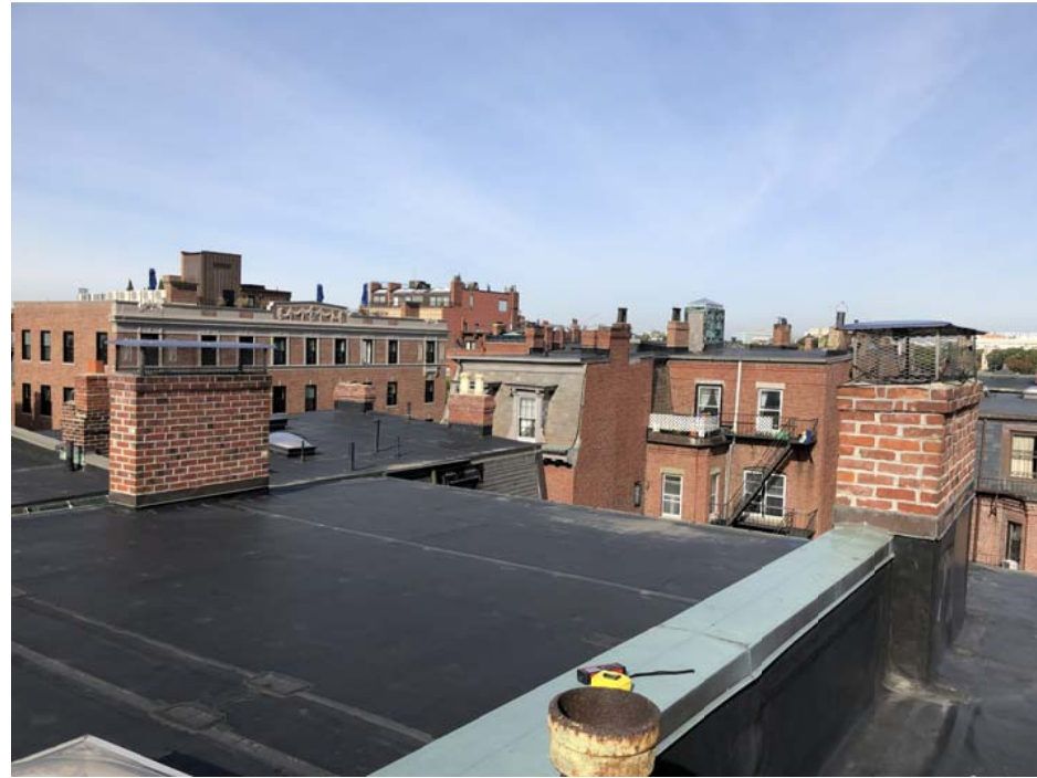
(A) Existing Condition - Roof looking Northwest
