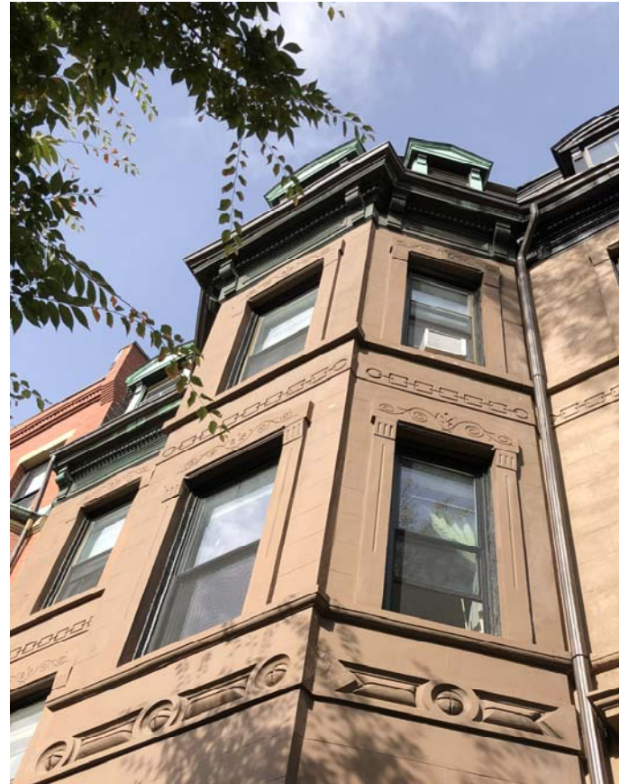
Example of Original Detail at 177 Marlborough
