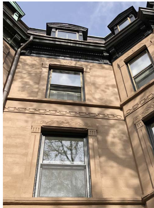
Example of Original Detail at 175 Marlborough
