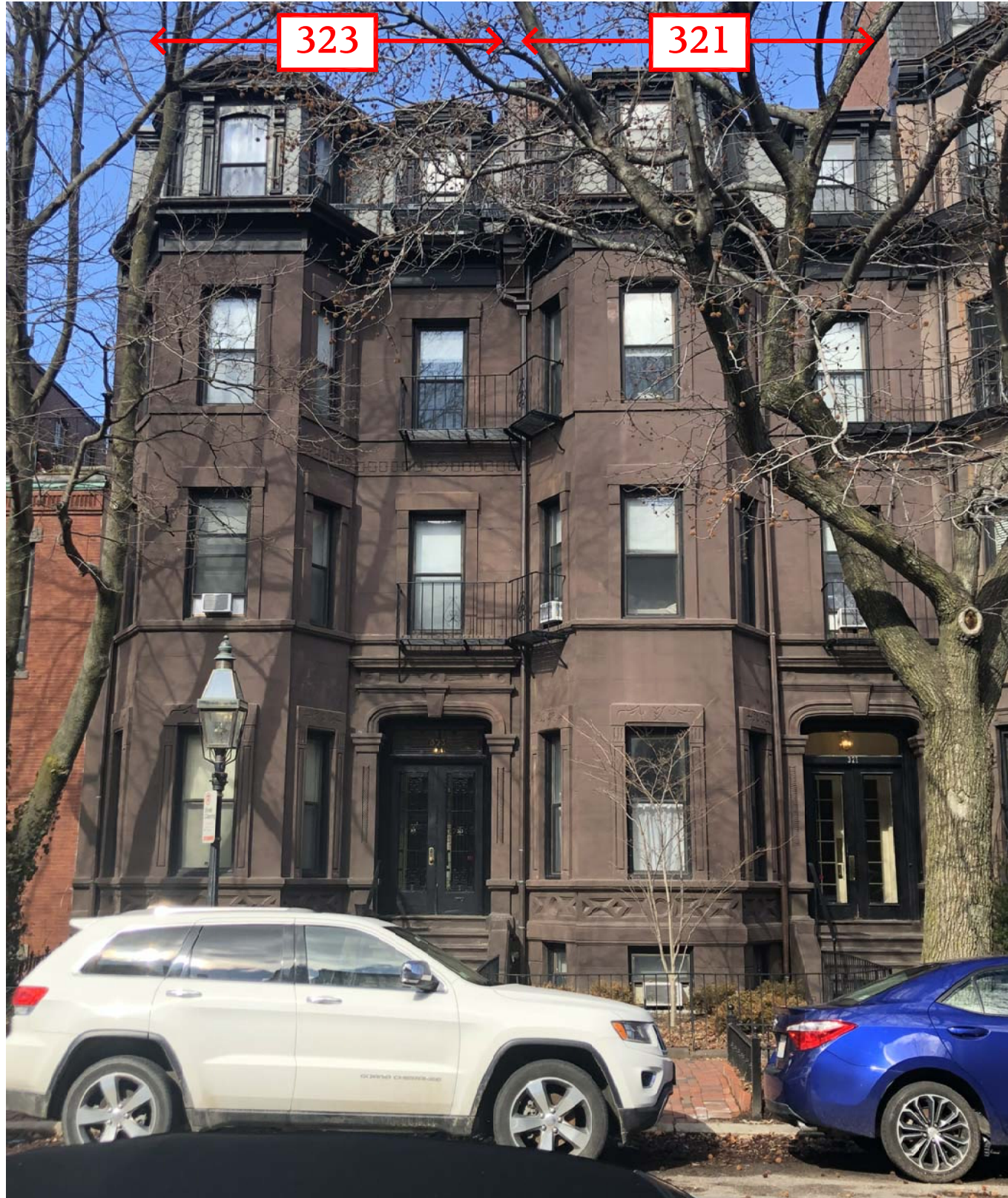
PHOTO "C" - Facade Elevation
