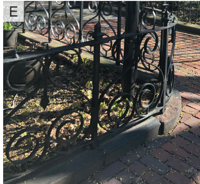
Existing Fence at 323
