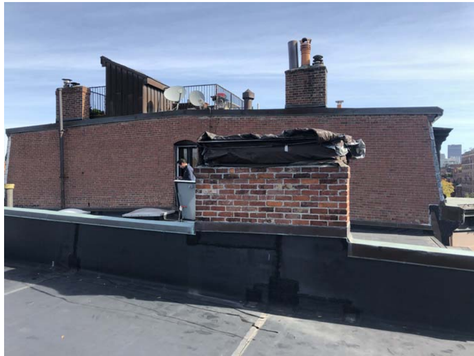
(G) Existing Condition - Roof looking West
