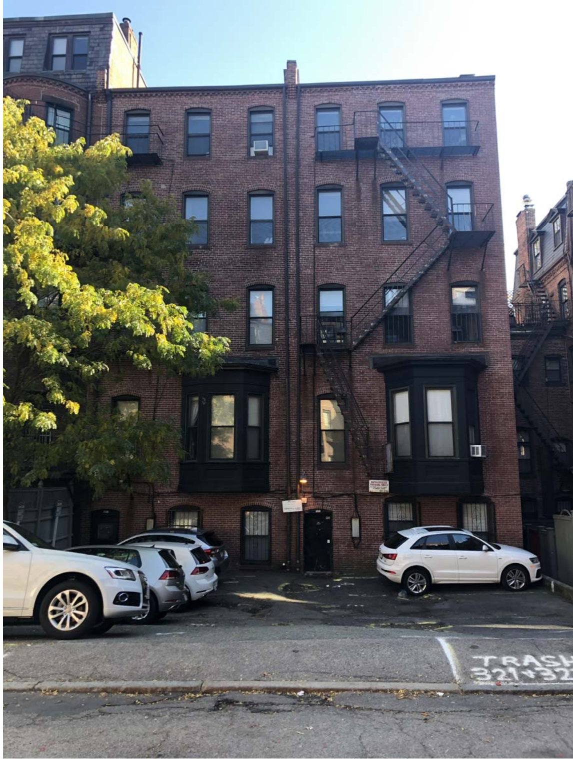
Existing Condition Public Alley Facade
