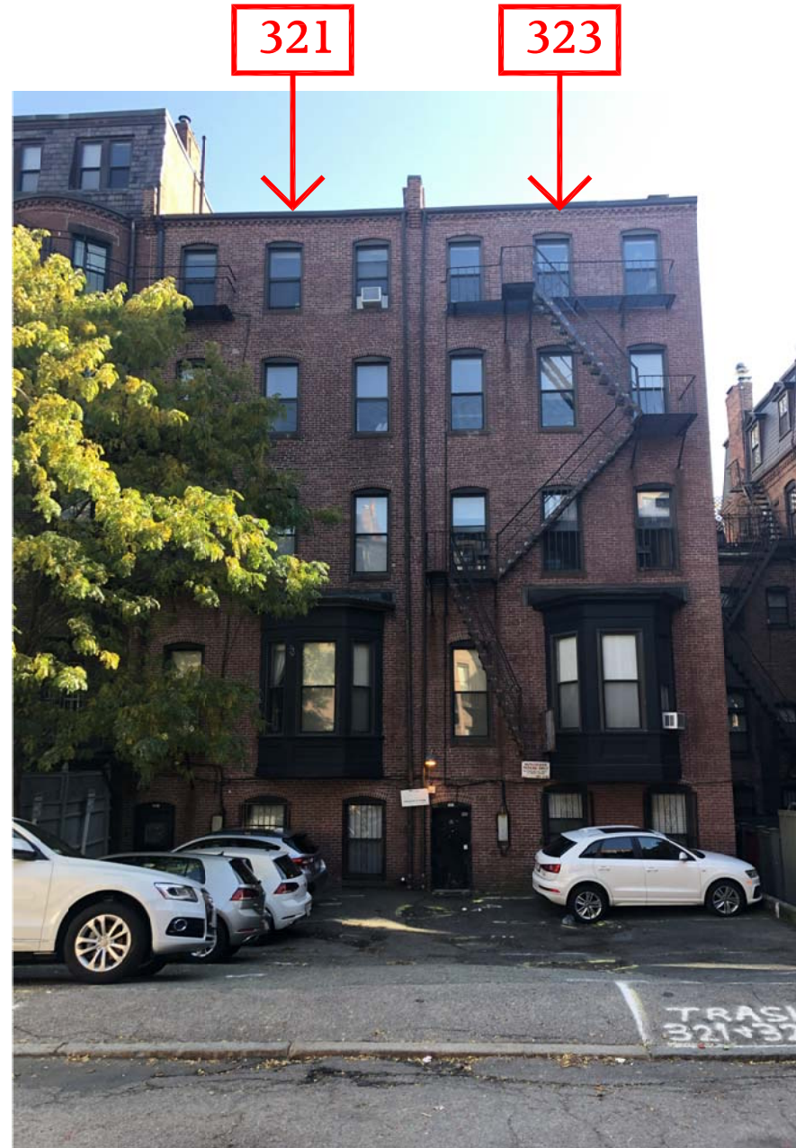
PHOTO "E" - Rear Facade
