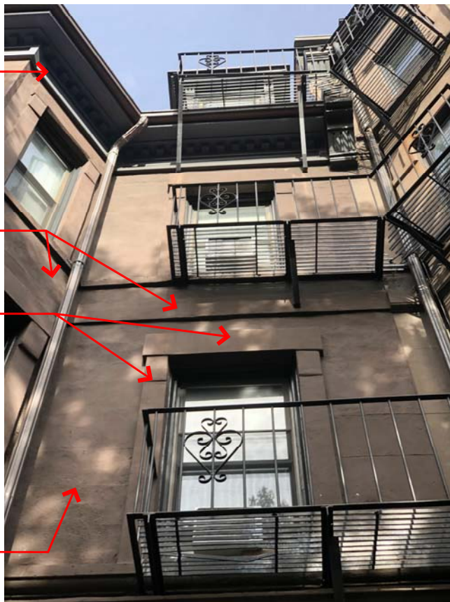
Existing Condition at 321 Marlborough
