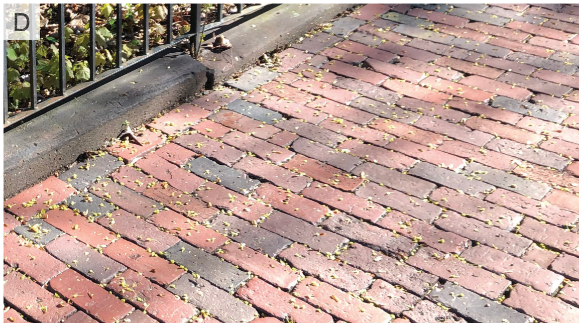
Existing Brick Paving
