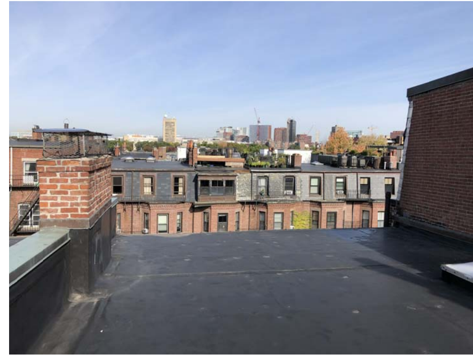
(B) Existing Condition - Roof looking North
