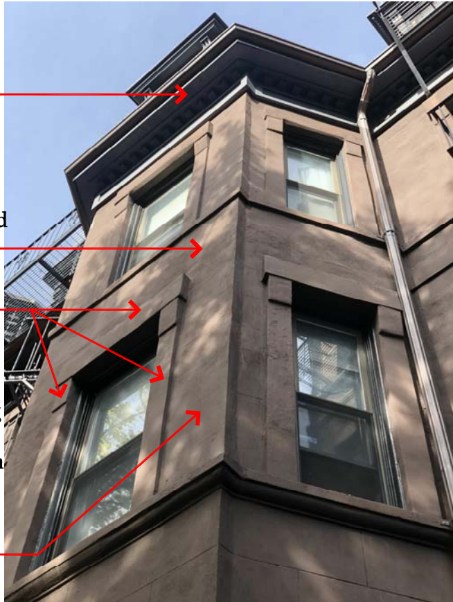
Existing Condition at 321 Marlborough
