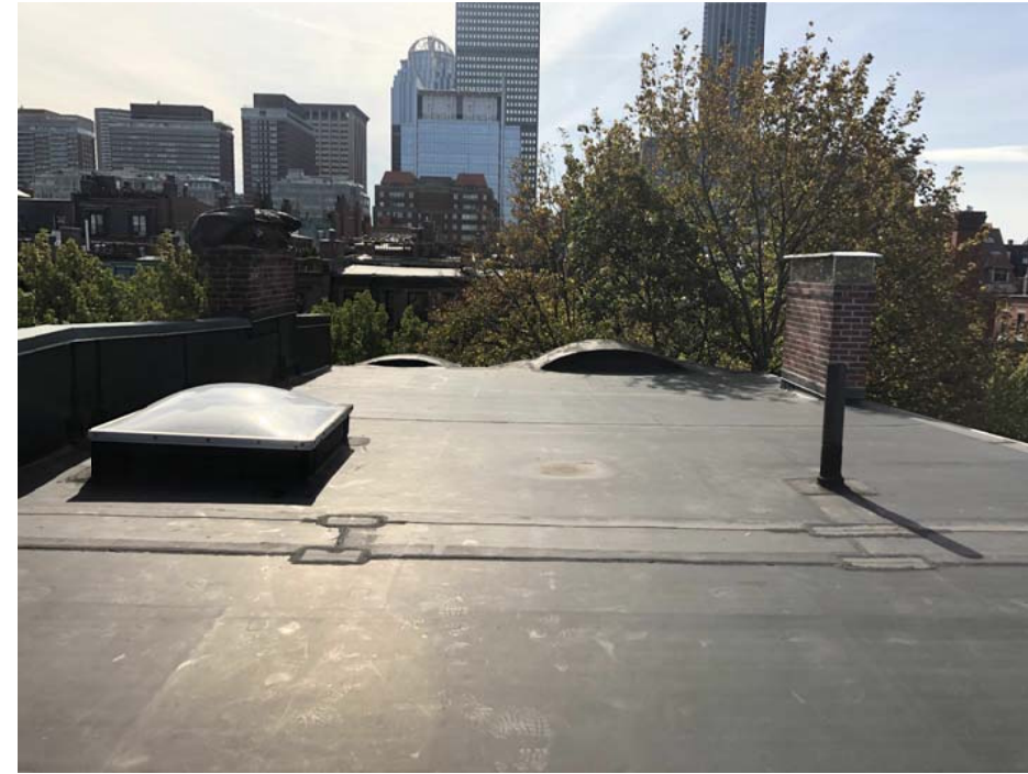
(F) Existing Condition - Roof looking South
