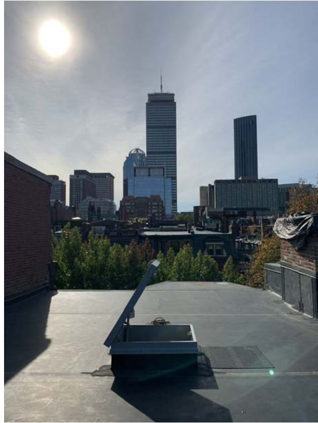
(E) Existing Condition - Roof looking South
