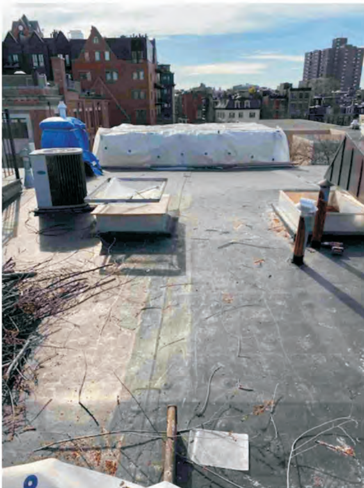
81 Warren Avenue Roof 3-9-2020
