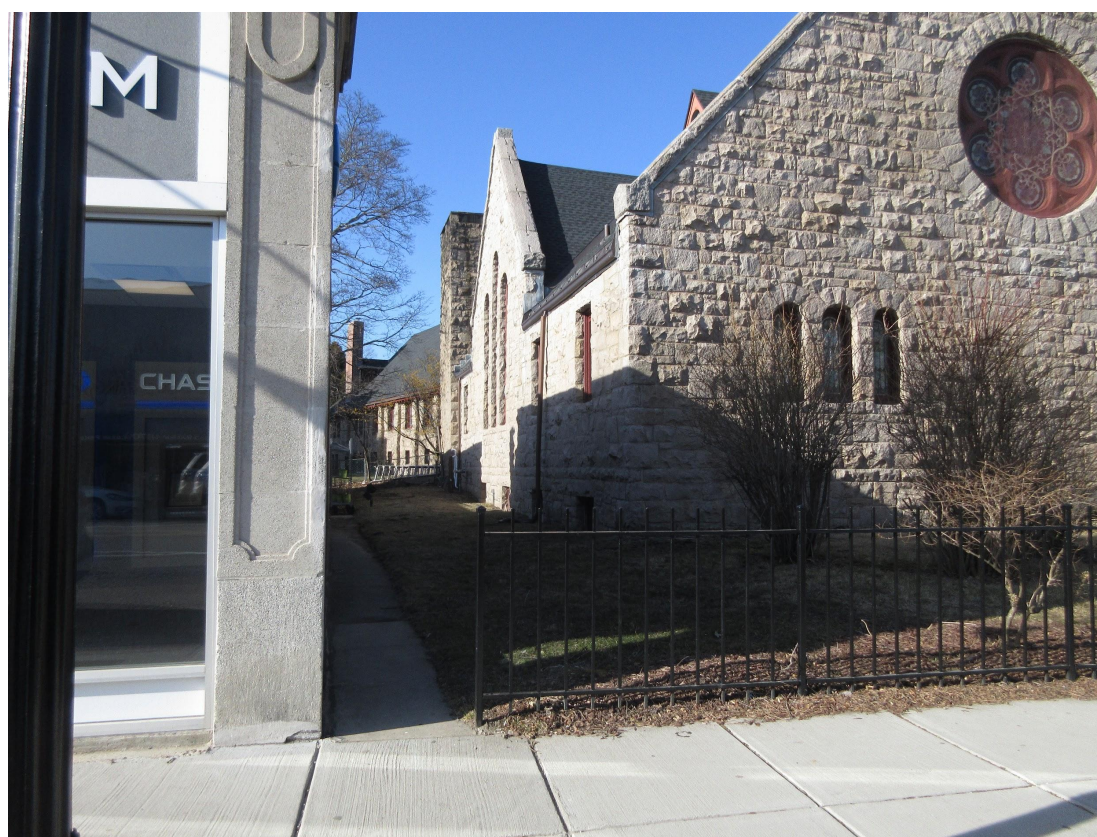
Current condition: alleyway from 1859 Centre St. sidewalk
