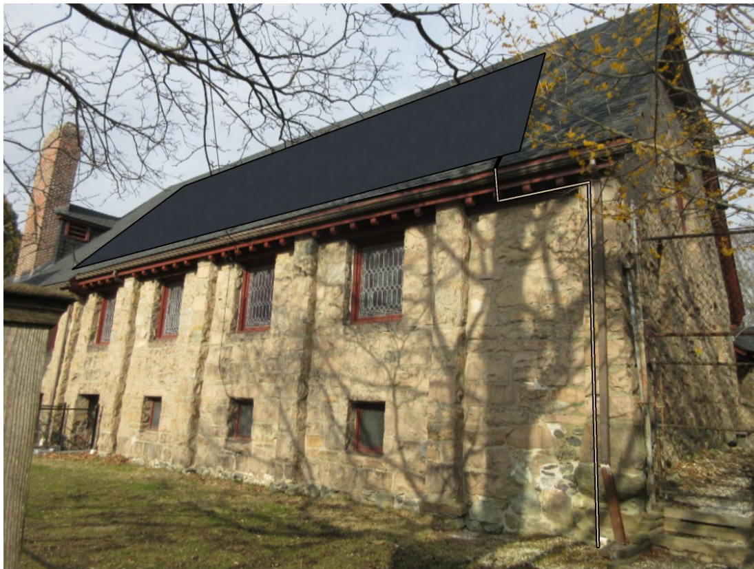
Parish Hall (70 Corey St.) roof from backyard with mock-up of solar panels and conduit
