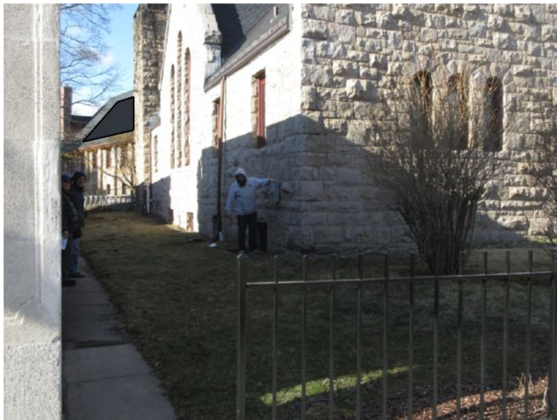
Mock-up view: alleyway from 1859 Centre St. sidewalk showing meter and cutoff switch location and solar panels on Parish Hall roof
