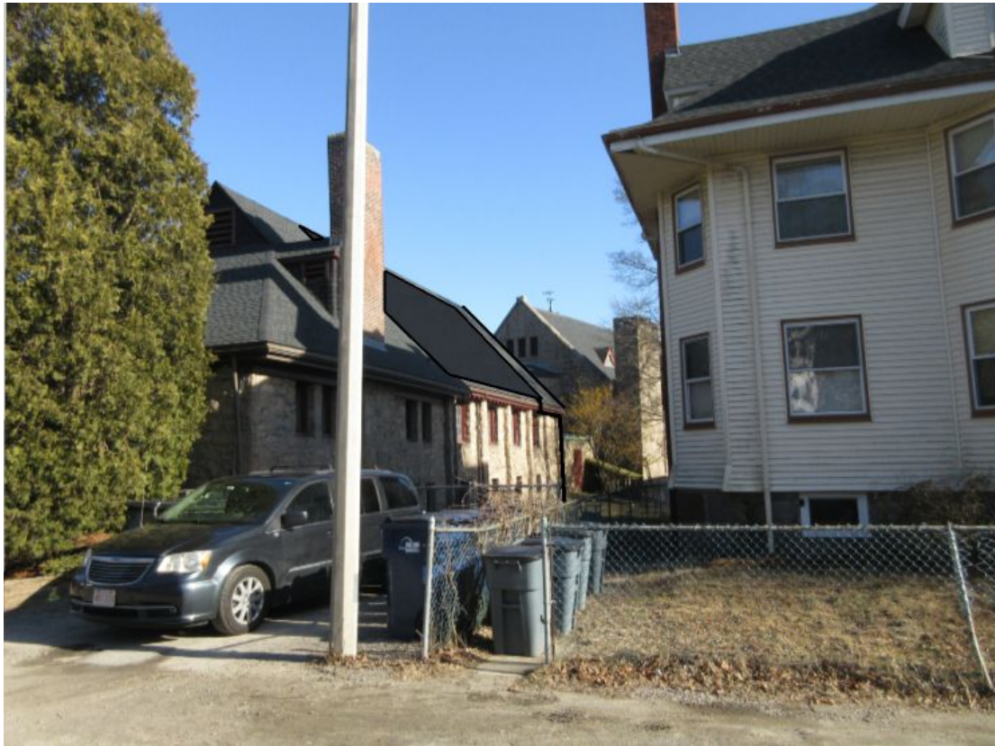
View of rear of Parish Hall (70 Corey St.) roof from Henshaw Terrace with mock-up of solar panels
