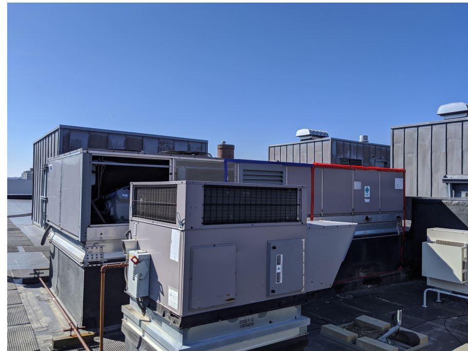
UNIT 2 EAST: View towards Necco Street
