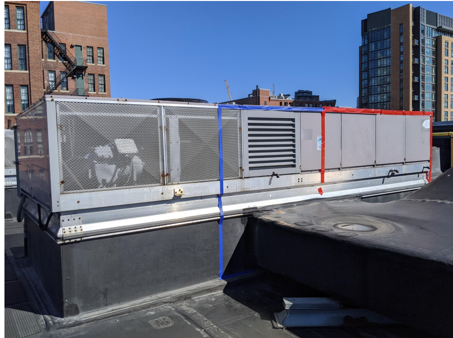
UNIT 2 WEST: View towards Necco Court and A Street
