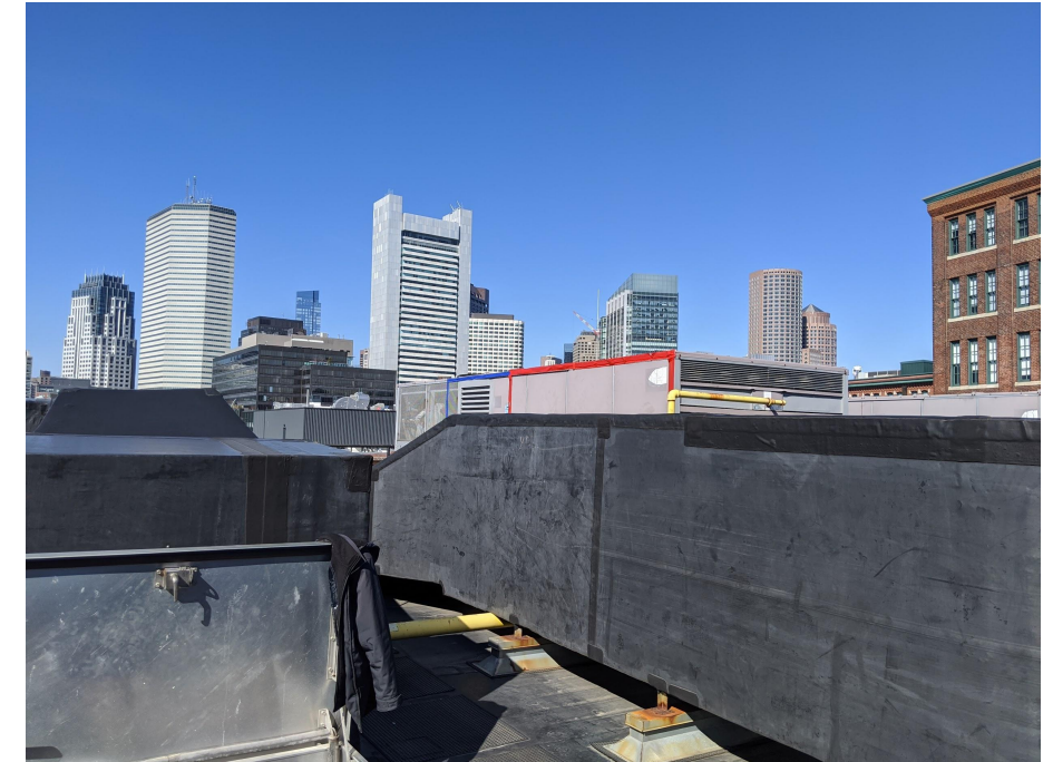
UNIT 2 WEST: View towards Atlantic Ave & Summer Street
