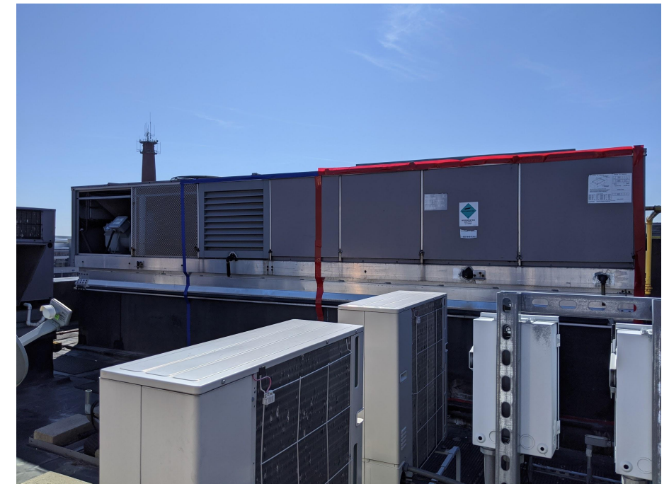
UNIT 2 EAST: View towards Necco Street.
