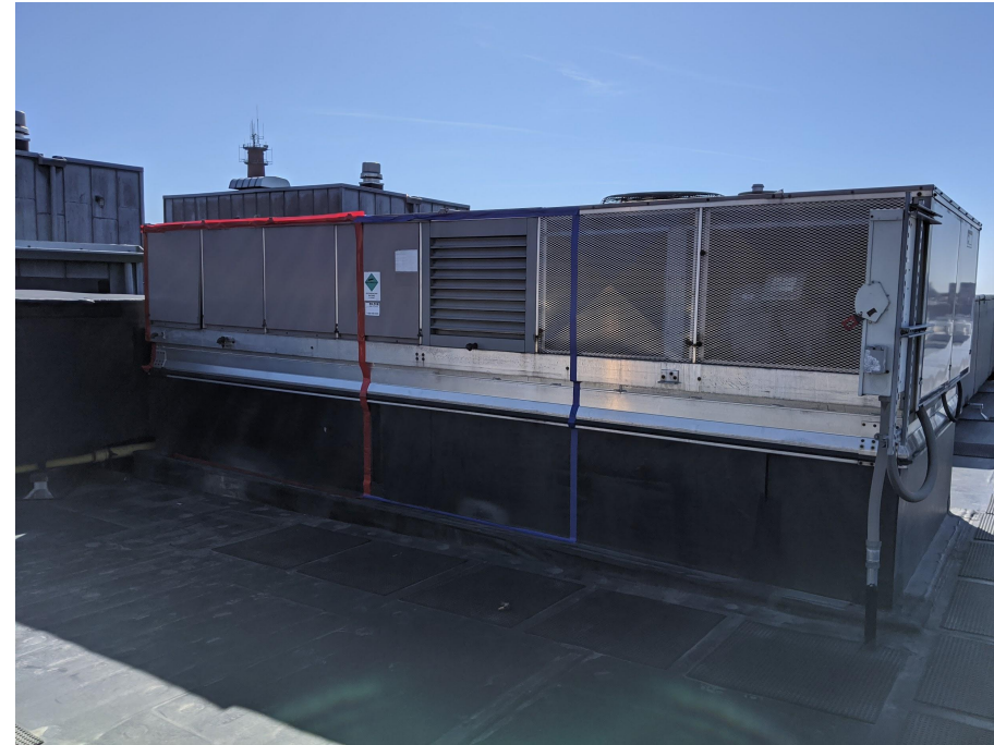
UNIT 2 WEST: View towards Necco Street
