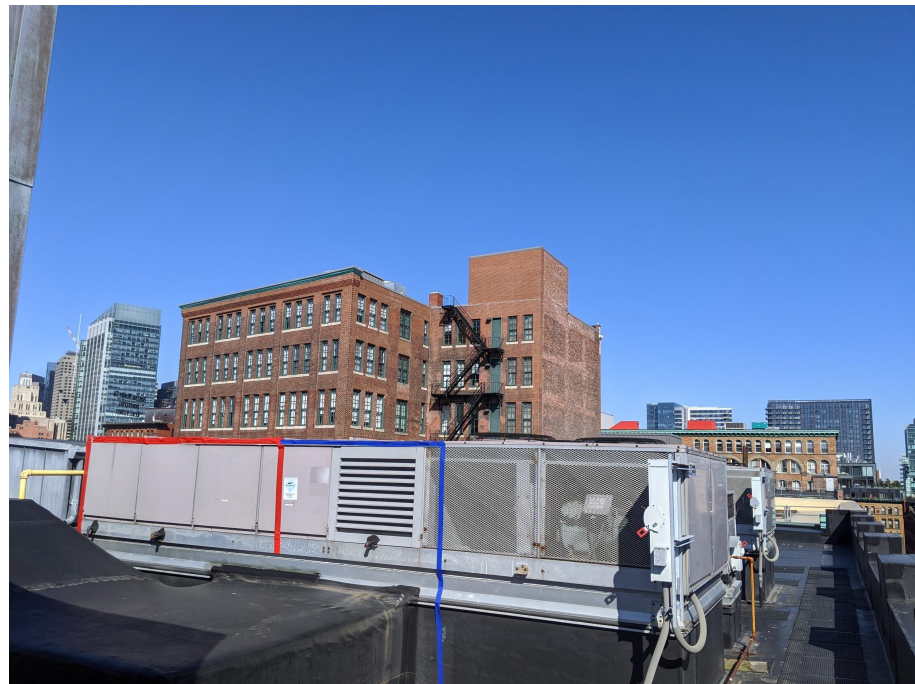
UNIT 2 EAST: View towards Necco Court
