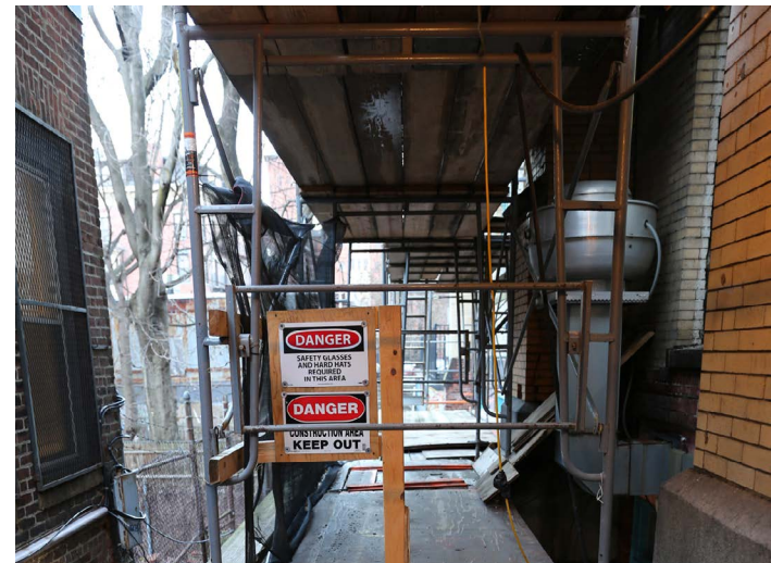
Protective scaffolding in alleyway (Spring 2019)
