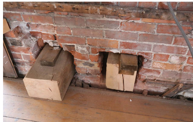
Exterior wall probes and temp support (Spring 2019)
