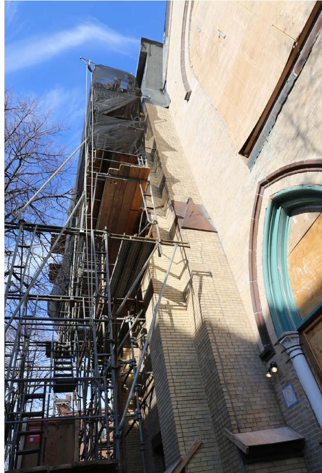
Scaffolded tower base (Spring 2019)
