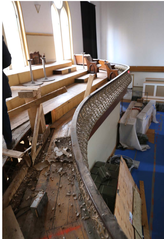
Existing balcony (Spring 2019)
