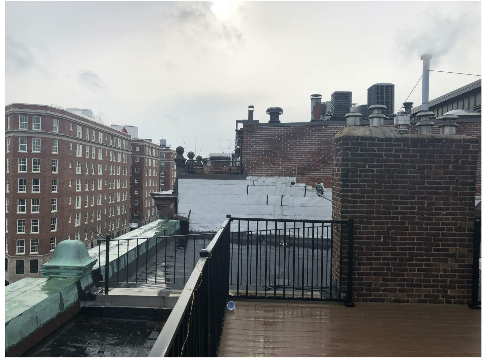
EXISTING ROOF DECK AT 7 BAY STATE ROAD - LOOKING TOWARDS KENMORE
