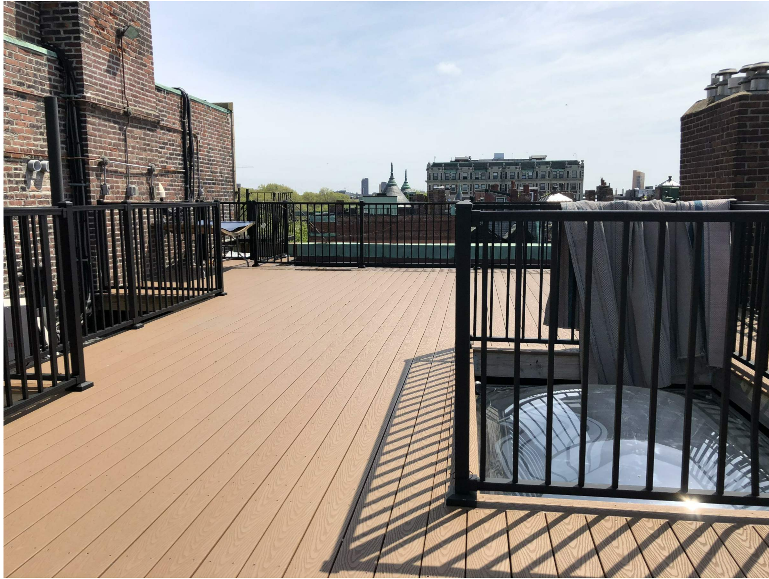
EXISTING ROOF DECK AT 7 BAY STATE ROAD
