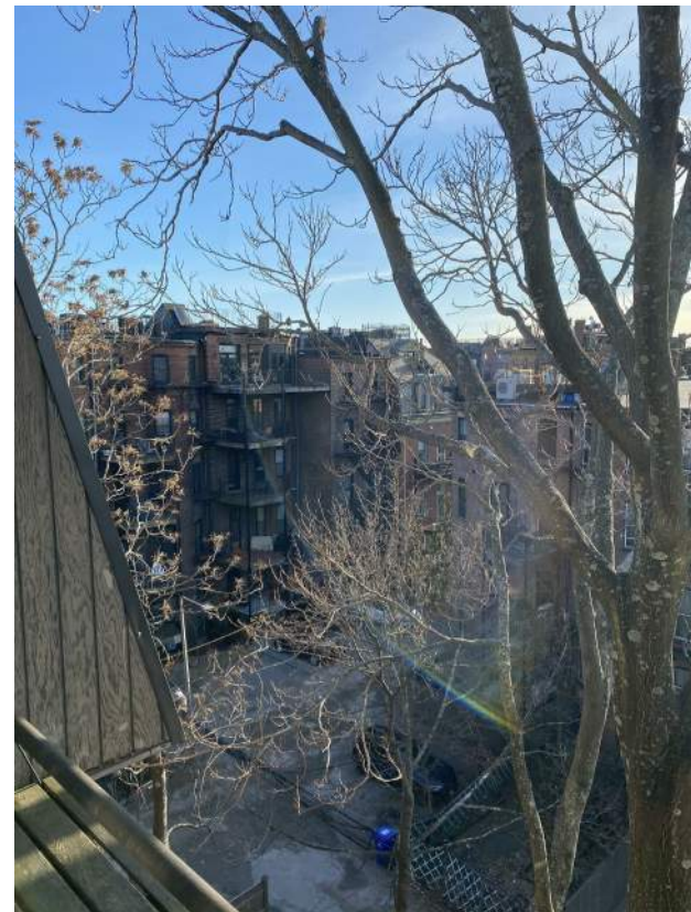
EXISTING PATIO AT MANSARD ROOF
