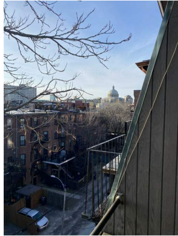
EXISTING PATIO AT MANSARD ROOF
